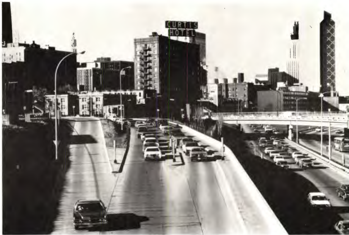
FIGURE 2. GRANT ST. BYPASS RAMP MERGE WITH 12TH ST. METERED RAMP
