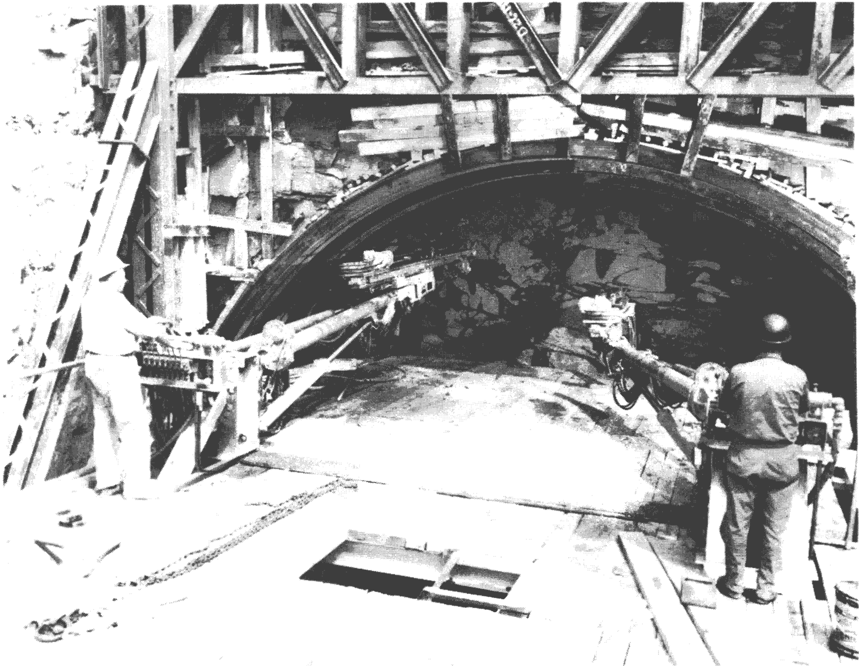
The conventional approach to rock tunnel excavation is the use of a drill jumbo. The photo shows tunnel workers on the top level of this three level equipment.
