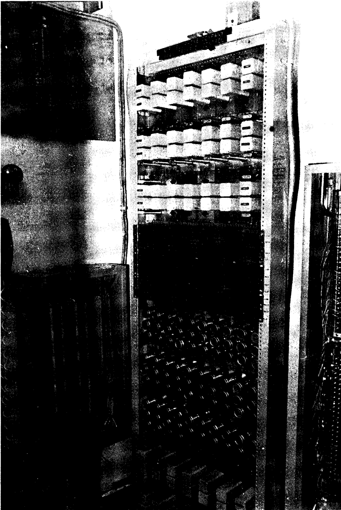
Figure 23. Telephone Termination Panel and Test Rack
