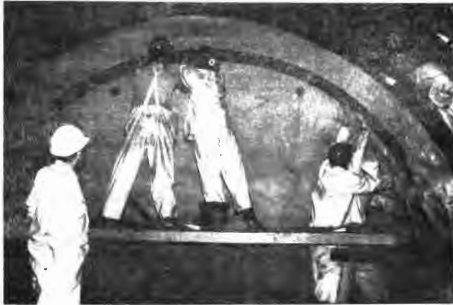
FIGURE 1-13 - INSTALLATION OF STEEL RING BEAMS
