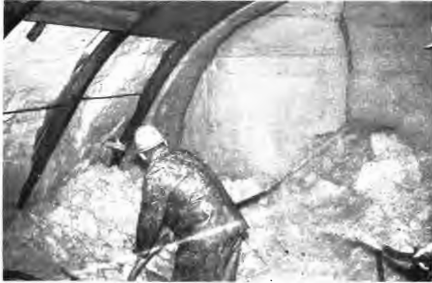
FIGURE 1-5 - SANDSTONE CUTTING WITH A HYDRAULIC LANCE
