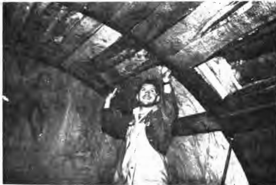
FIGURE 1-14 - INSTALLATION OF TIMBER LAGGING
