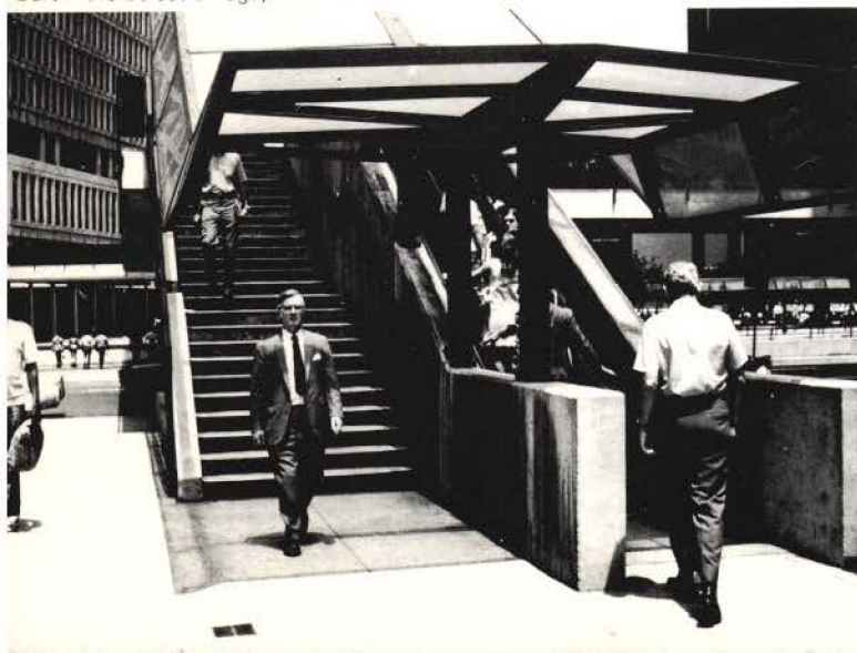
Baltimore Street Bridge, Baltimore
