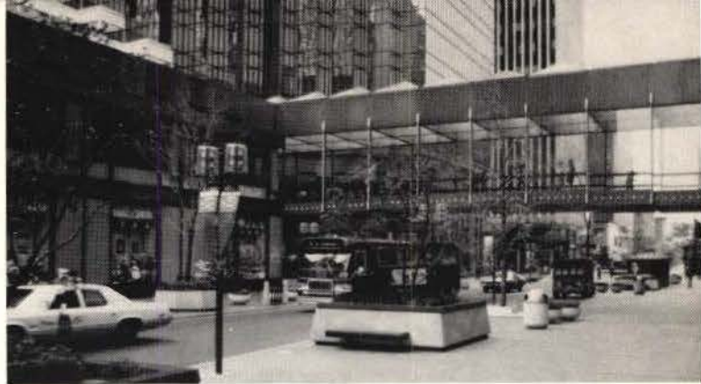
Skyway Bridge crossing Nicollet Mall, Minneapolis
