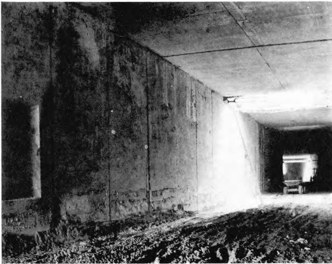
Fig. 51 Precast concrete wall panels before any finish is applied. (Courtesy Soletanche and Rodio, Inc.)
