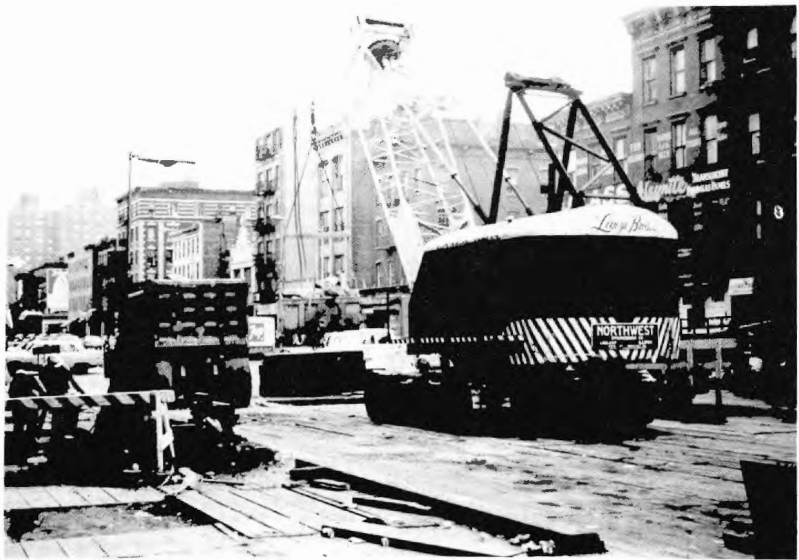
Fig. 31 Construction equipment and supplies causes temporary live loads on Cut-and-cover tunnel structures. system.
