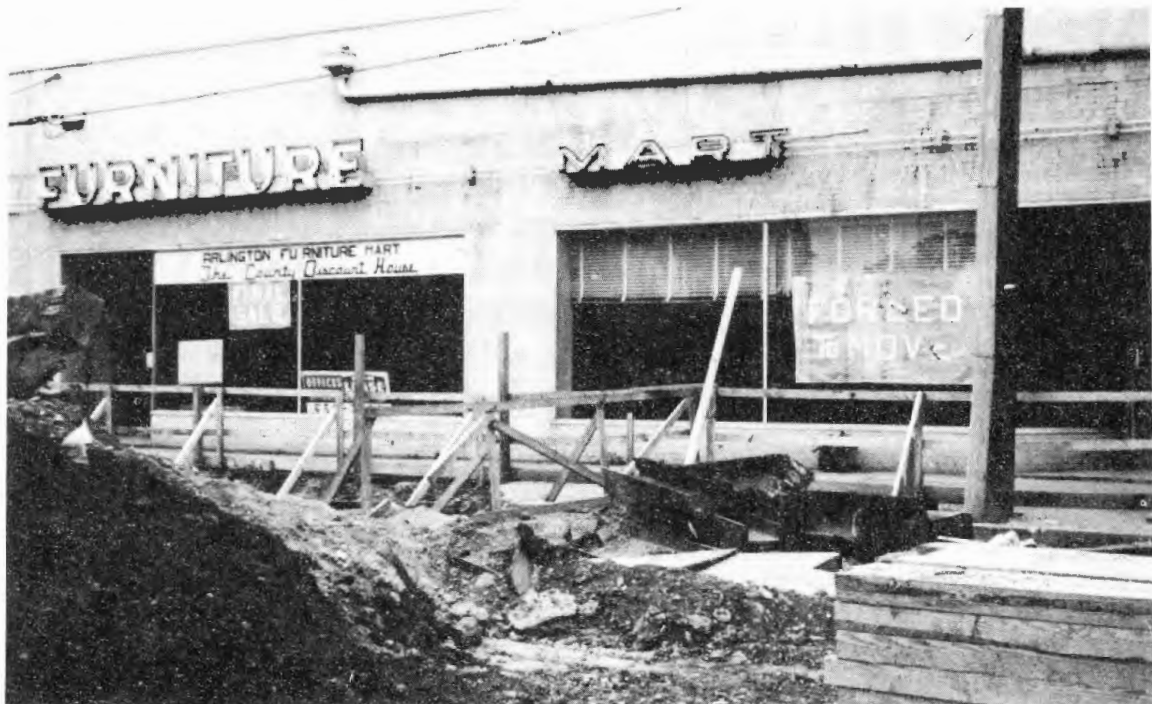
Fig. 2 Cut-and-cover tunnel construction may cause severe business disruption
