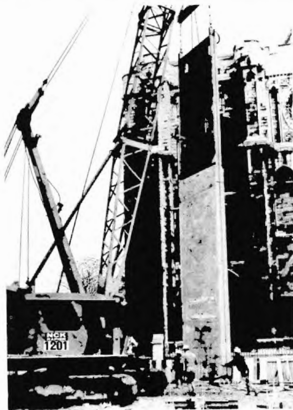
Fig. 7 Installing precast concrete wall panel in slurry trench. (Courtesy Soletanche and Rodio, Inc.)
