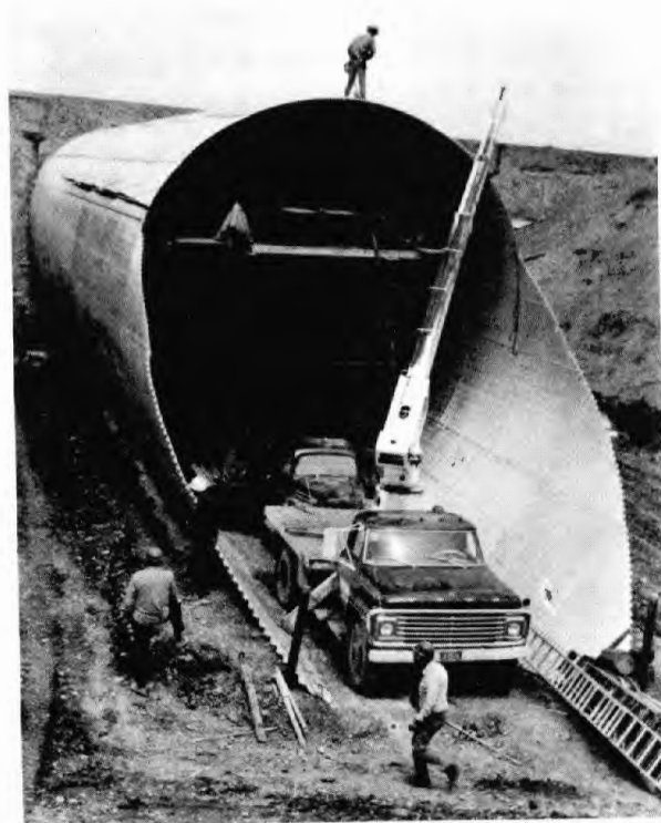
Fig. 4 Long span corrugated steel arch. (Courtesy Armco Steel Corporation)
