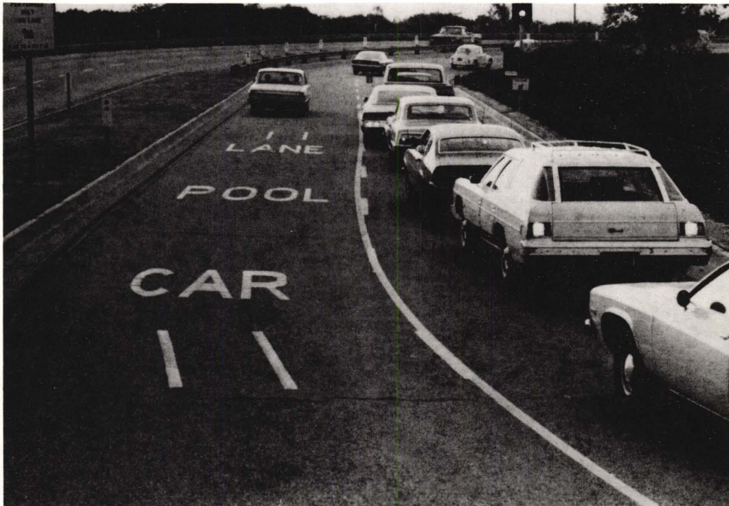
Figure 5. Bus and carpool bypass lane, Los Angeles.
