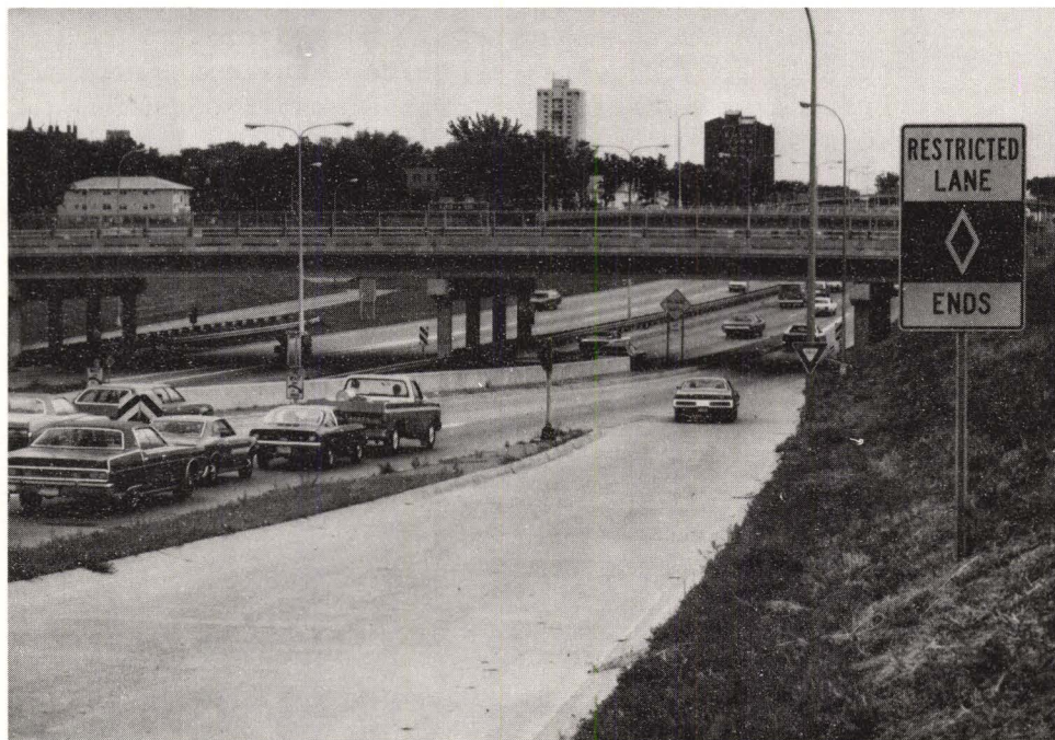
Figure 11. Grant Street ramp.
