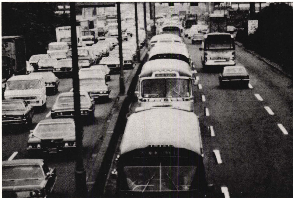
Figure 29. I-495 contra-flow bus lane to New York City.
