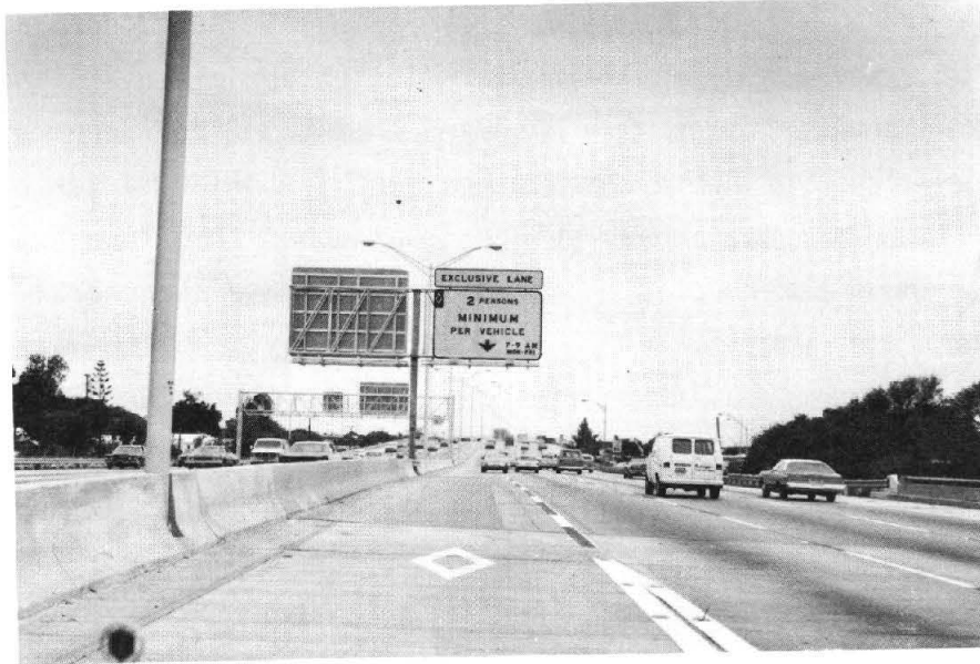
FIGURE 6.1. EXCLUSIVE LANE IDENTIFICATION SIGN MODIFIED FOR TWO PASSENGER CAR POOLS.
