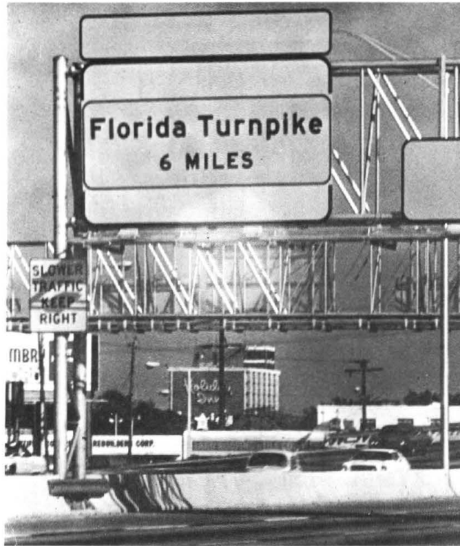
FIGURE 3.2. TEMPORARY REPLACEMENT OF "MISSING" EXCLUSIVE LANE SIGN AT LOCATION TWO.
