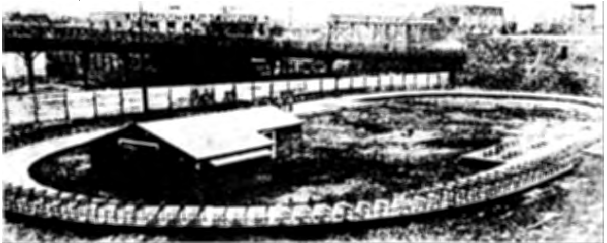
Full scale model in Jersey City of a 1924 Putnam Proposal for a three stage continuous loop system to replace the N.Y.C. Times Square Shuttle. Seats positioned on the high speed section.
