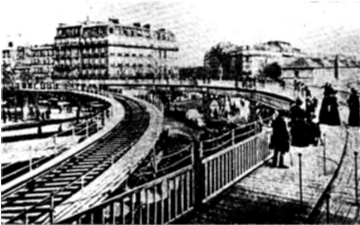
The moving platform installed at the 1900 Paris Exposition, photo illustrates low speed boarding and exiting stage at right, higher speed stage at left.
