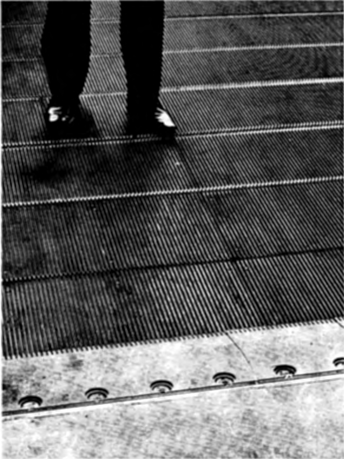
VIEW OF SPEEDAWAY EXIT ILLUSTRATING GROOVED PALLETS AND STATIONARY COMBPLATE.
