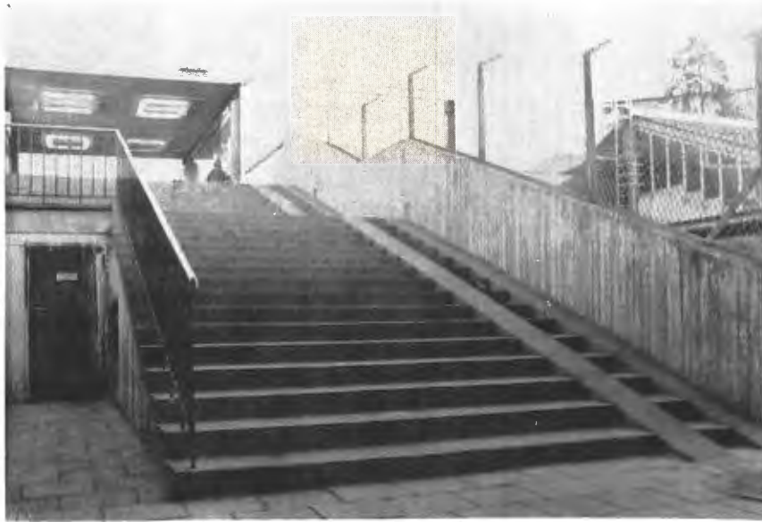
Dual track ramp incorporated in a concrete stairway.
