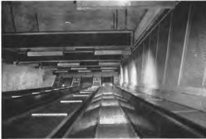
View from upper landing of escalator. Inclined elevator enclosure on right.
