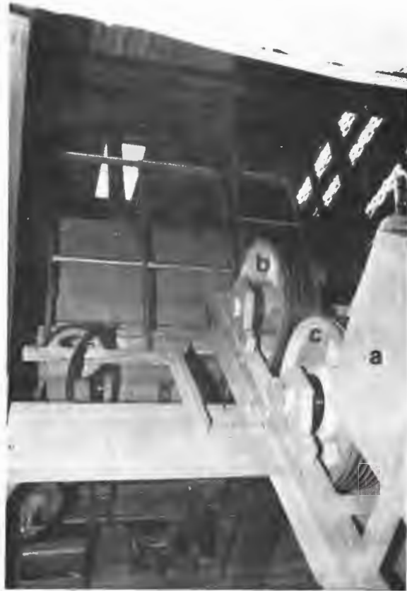
Hoist machine(a) and deflector sheaves for car(b) and counterweight(c) cables.
