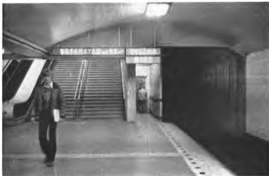
Train room landing of vertical elevator, separated from foot of escalator and stairway, at end of short corridor.
