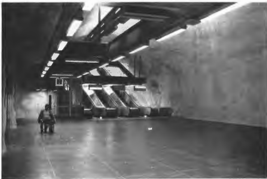
Train room landing of mesh- and glass-enclosed inclined elevator, coinciding with escalator landing. A member of the study team is at left.
