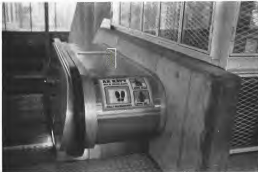
Fare hall landing approach to escalator and inclined elevator.
