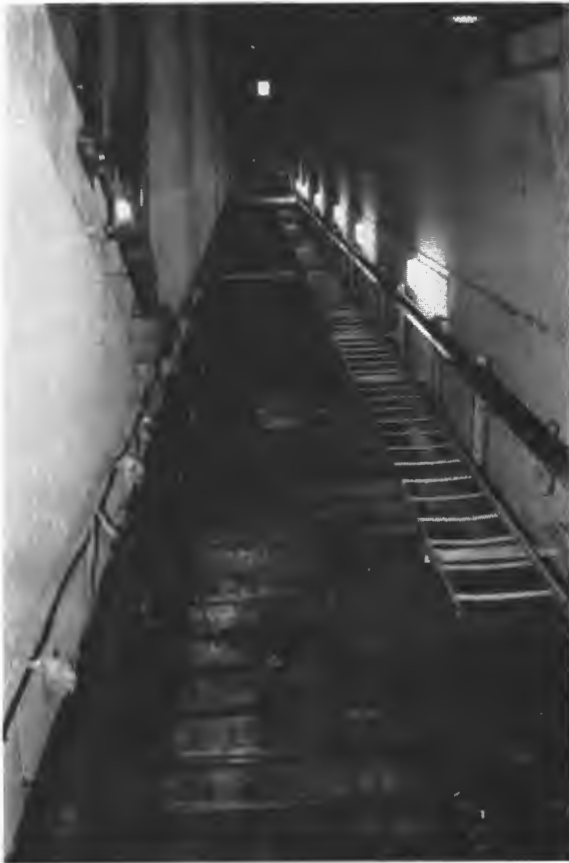
View of inclined elevator shaft, looking upward toward car.
