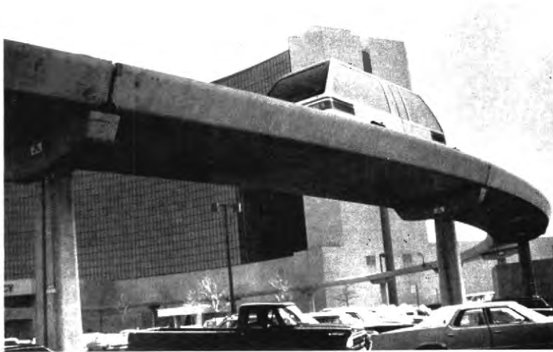
(a) Fairlane AGT System Guideway-Dearborn, Michigan
