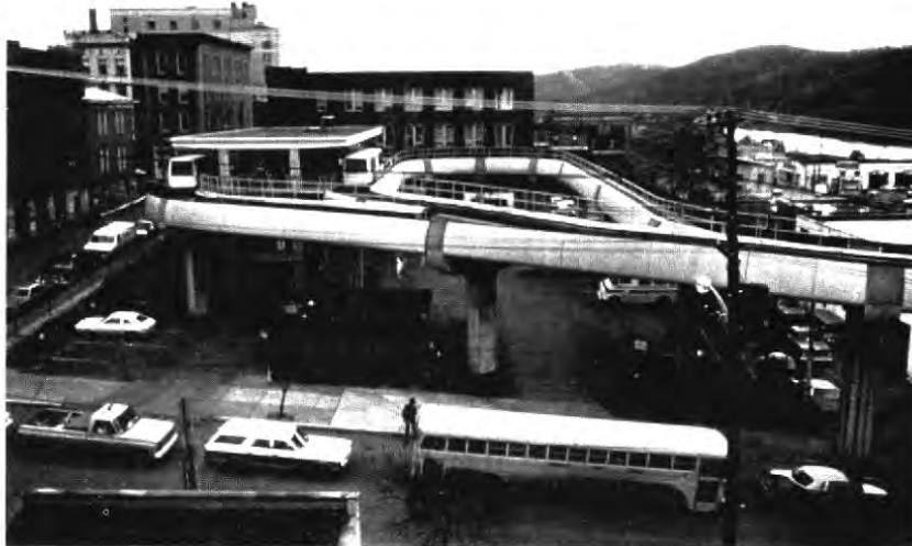
(a) Walnut Street Station, Morgantown AGT System Morgantown, West Virginia
