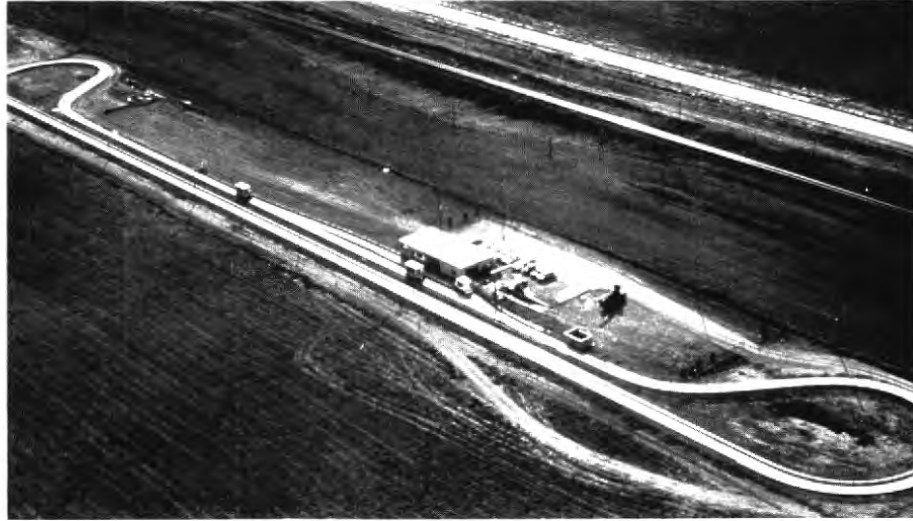
a) Otis Test Facility, Denver, Colorado Straight Section, 513 Meters Long; Curved Sections, 257 Meters Long; Station Siding, 88 Meters Long
