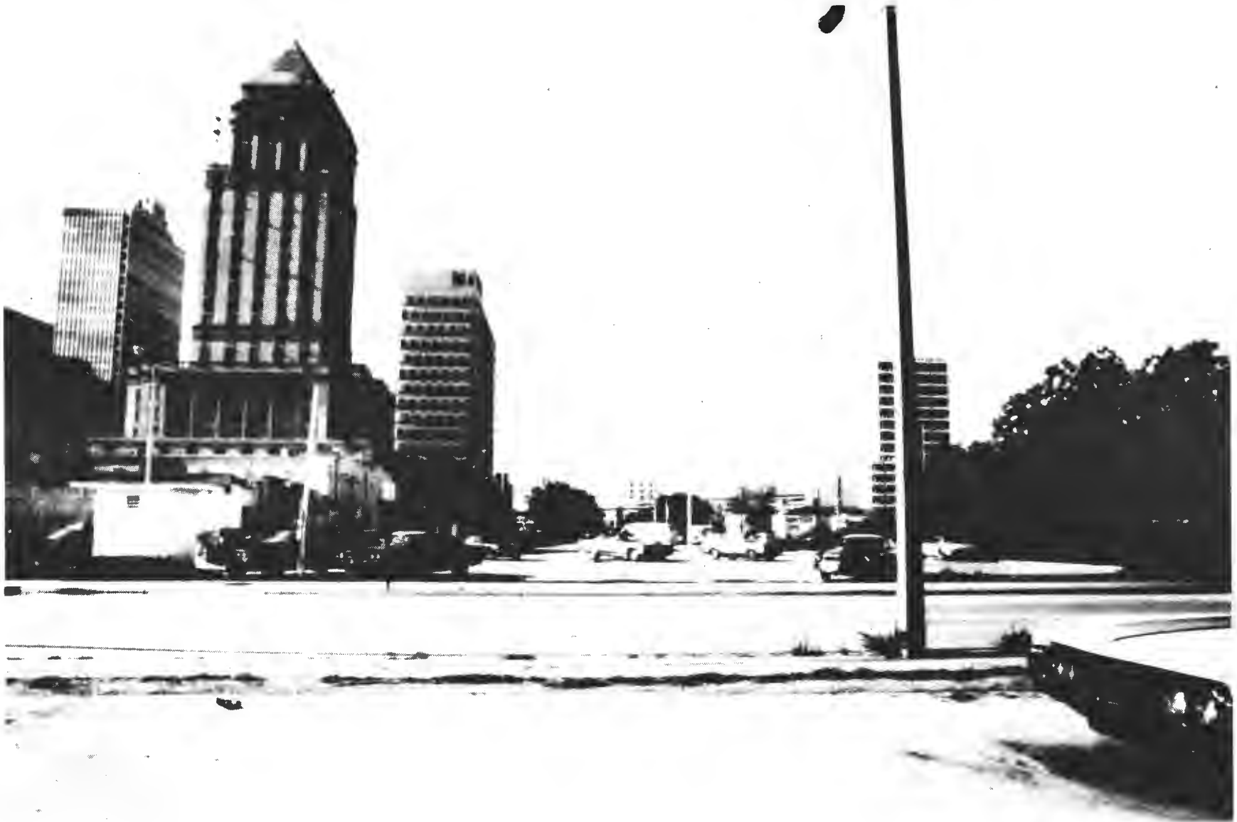
EXISTING GROUND LEVEL VIEW OF COURTHOUSE FROM NORTH
