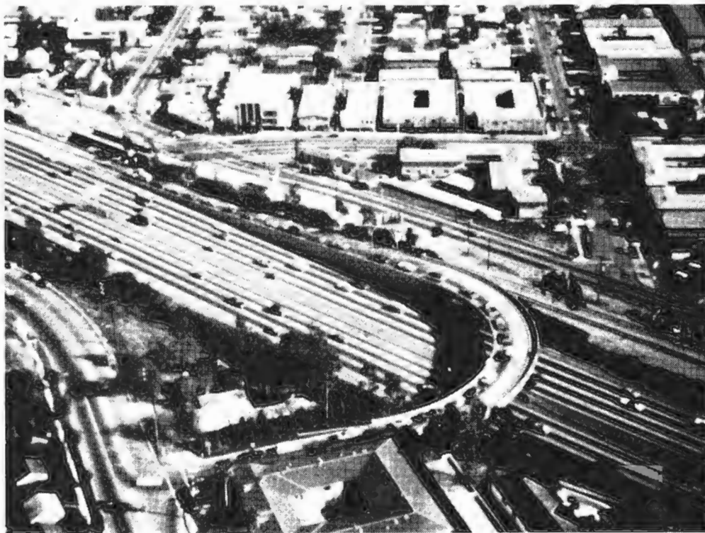
Autos Waiting at Metered On-ramp with Bypass Lane for Buses and Carpools, Santa Monica Freeway, California
