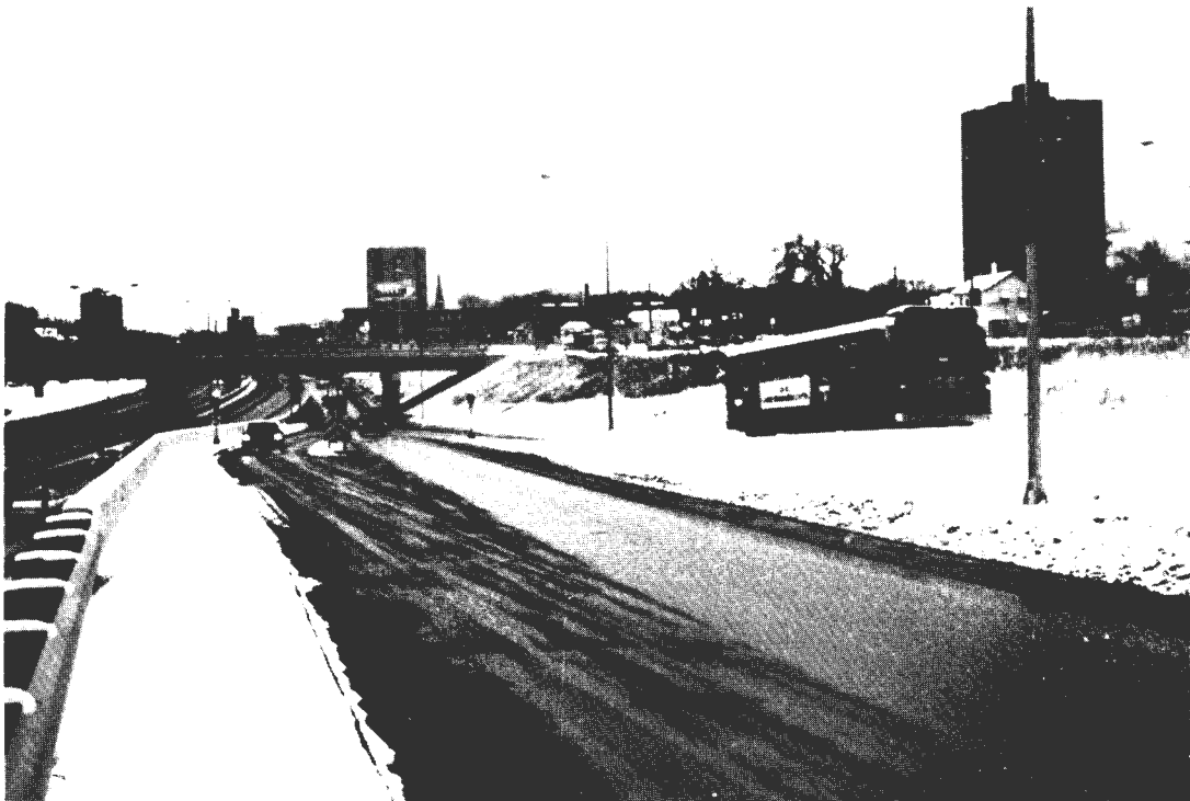
Minneapolis I-35W: Metered Ramp with Bypass Lane for Express Buses
