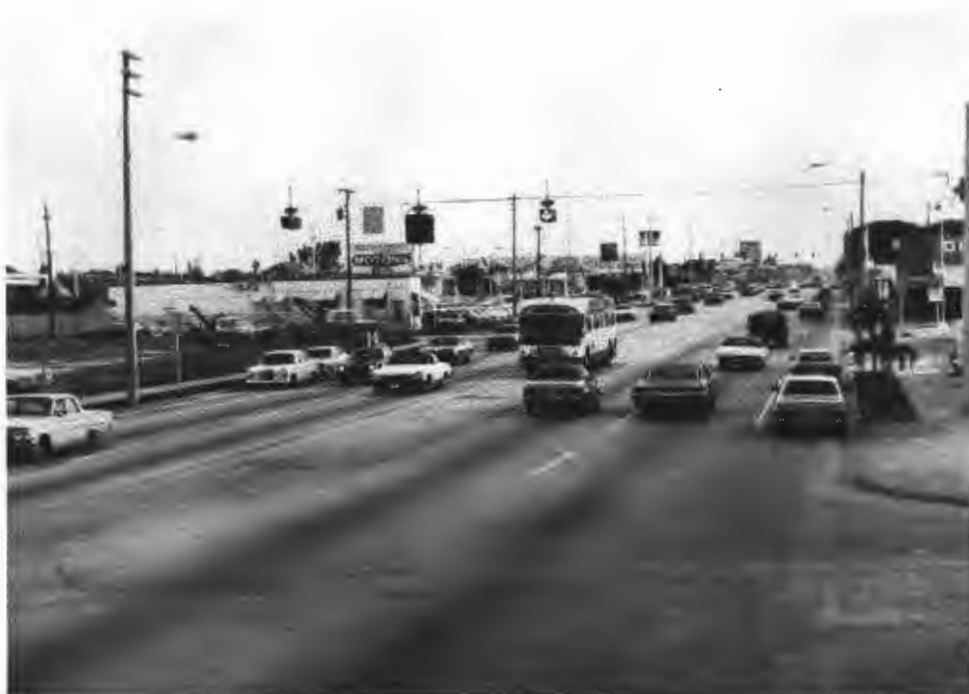
Reversible Reserved Bus Lane with Traffic Signal Preemption; N.W. 7th Avenue, Miami, Florida
