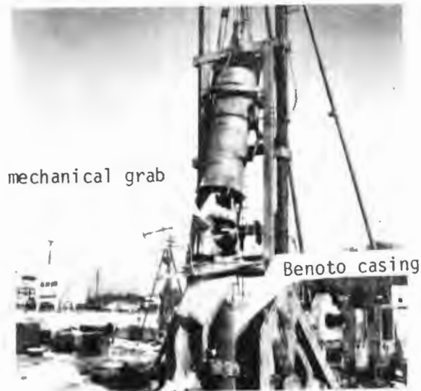
Figure 3.15 Benoto Rig
