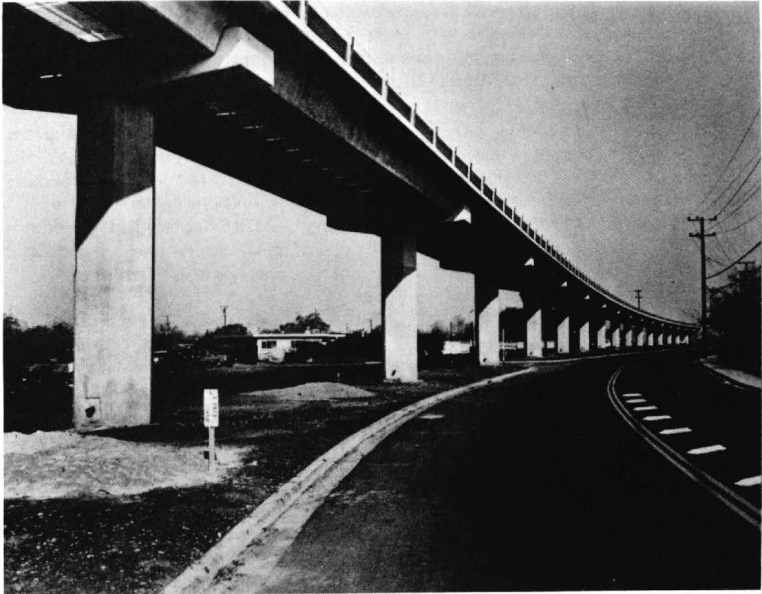
PLATE III-3 AERIAL LINE CONSTRUCTION, WALNUT CREEK
