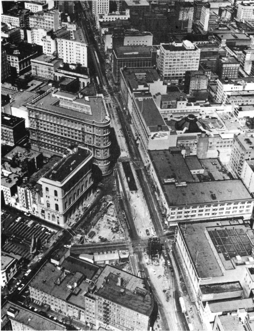
PLATE III-1 CUT-AND-COVER CONSTRUCTION, DOWNTOWN SAN FRANCISCO
