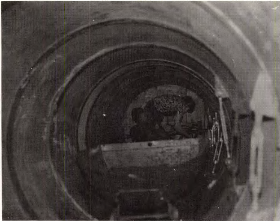
PLATE AIV-10. Heading of pipe jacking operation for station roof
