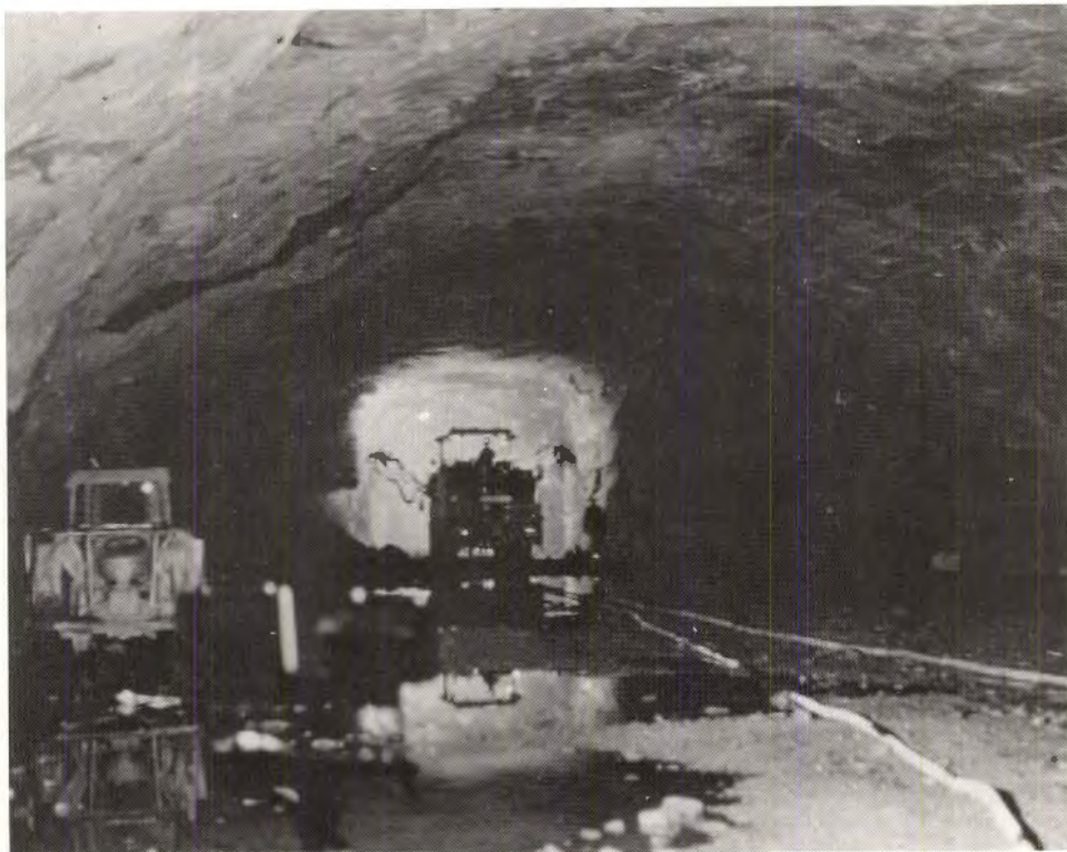
PLATE AIV-26. Top heading of Brofjorden oil storage chamber
