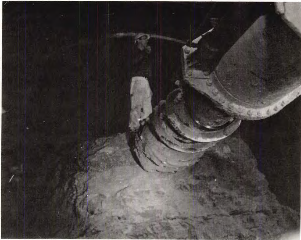
PLATE AIV-15. Excavation of top heading
