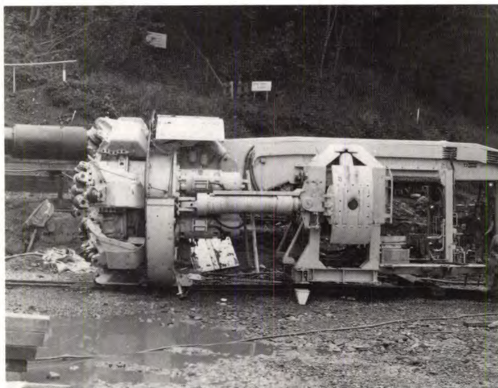
PLATE AIV-2. Robbins TBM; note open working space behind cutter head for support installation
