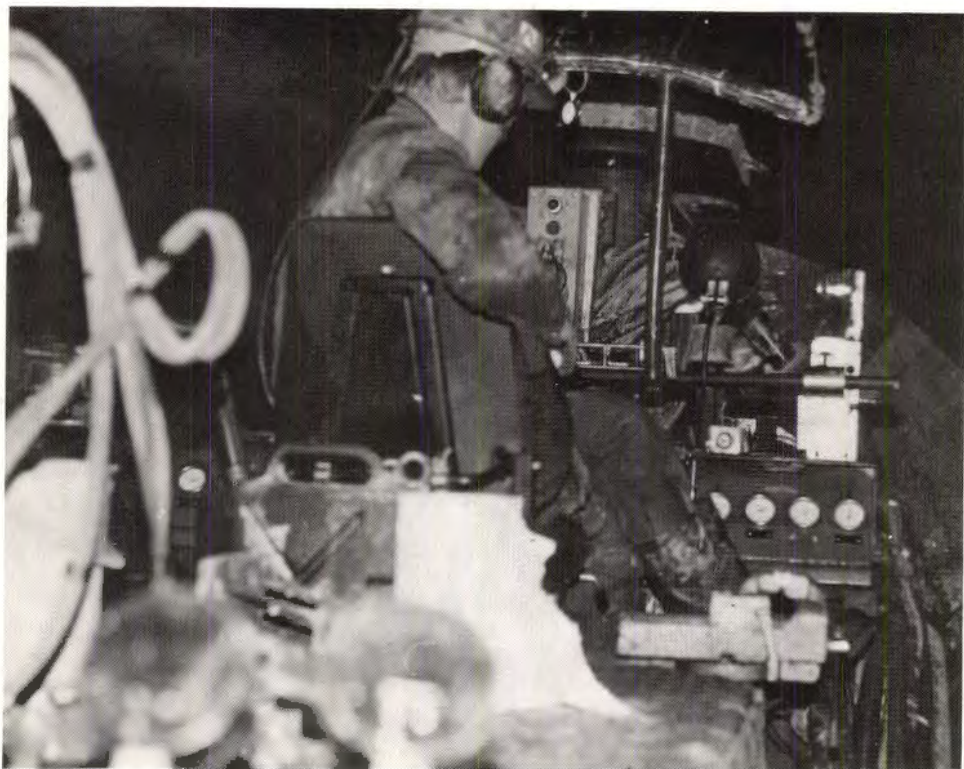
PLATE AIV-21. Bouygues TBM
