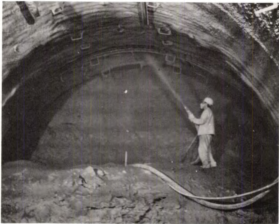
PLATE AIV-16. Application of shotcrete to top heading
