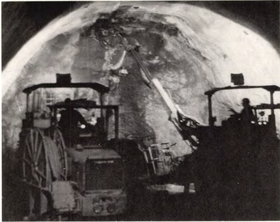
PLATE AIV-23. Drilling for next round
