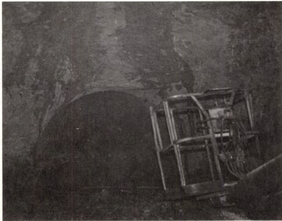
PLATE AIV-24. Pilot tunnel near invert of main heading
