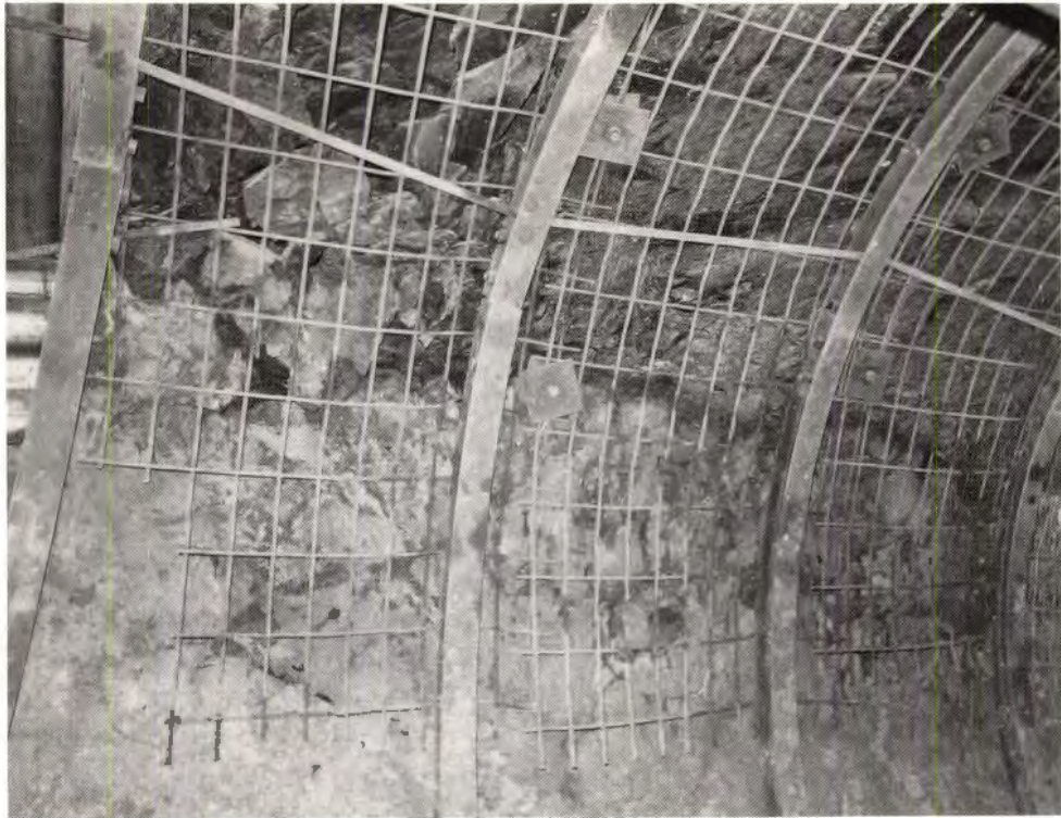
PLATE AIV-8. Shattered mudstone (top) and friable sandstone (bottom), Tees station 4300
