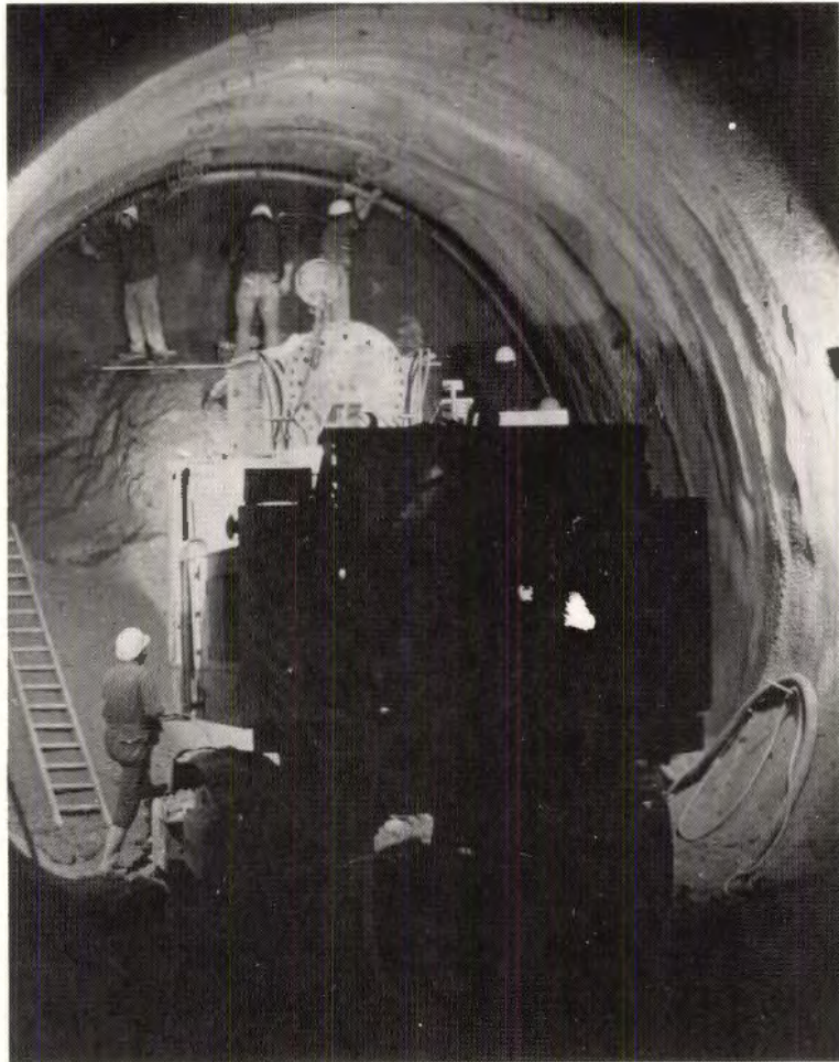
PLATE AIV-14. Demag roadheader at tunnel face
