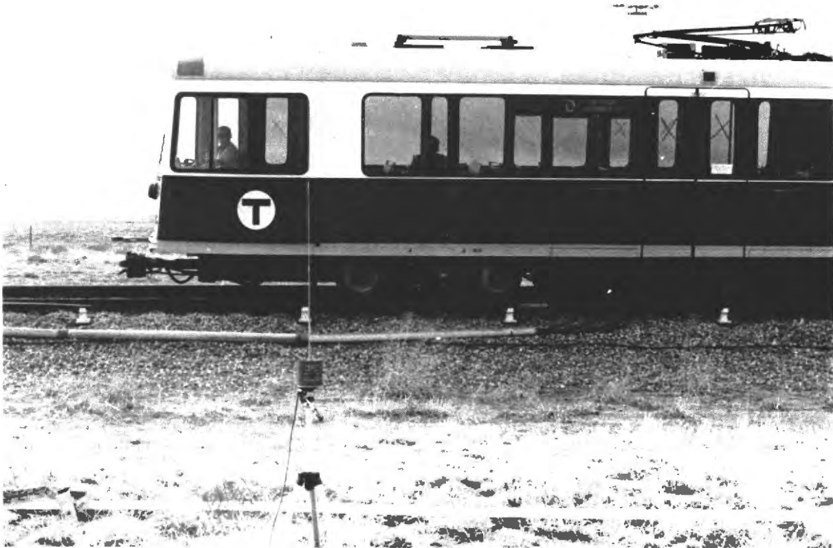
Figure 4-3. Typical Wayside Antenna Installation
