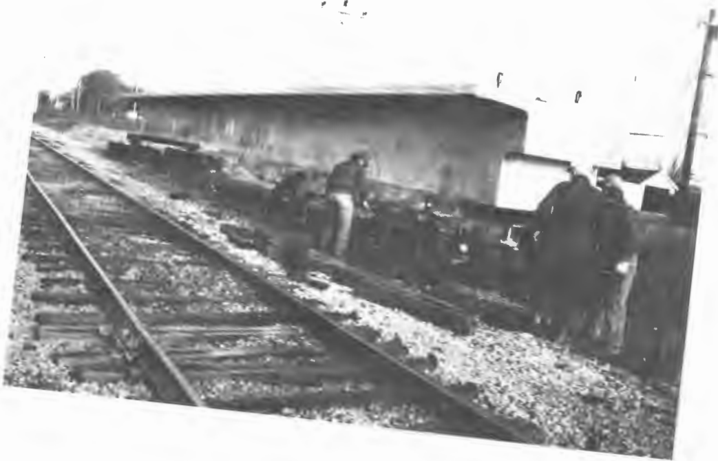
Fig. 3 Transportation of Girders by Railroad
