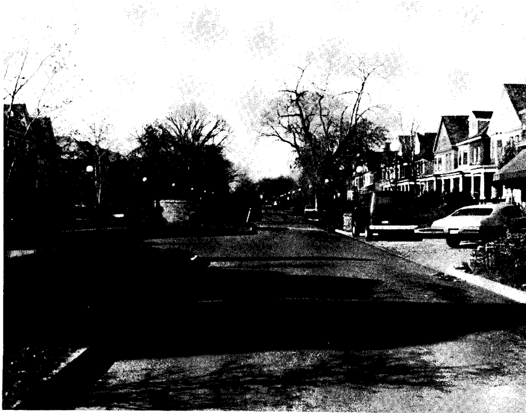
Laclede Street, showing median strip and ball-and-chain closing. (Photo courtesy St. Louis Department of Streets.)
