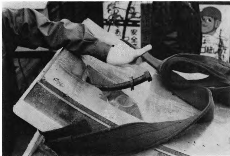
Figure 13. PRECAST CONCRETE LINER SEGMENTS: UPPER PHOTOGRAPH, CONVENTIONAL SEGMENTS WITH GROOVES FOR WATERPROOFING: LOWER PHOTOGRAPH, SEGMENTS WITH CURVED BOLT HOLES.
