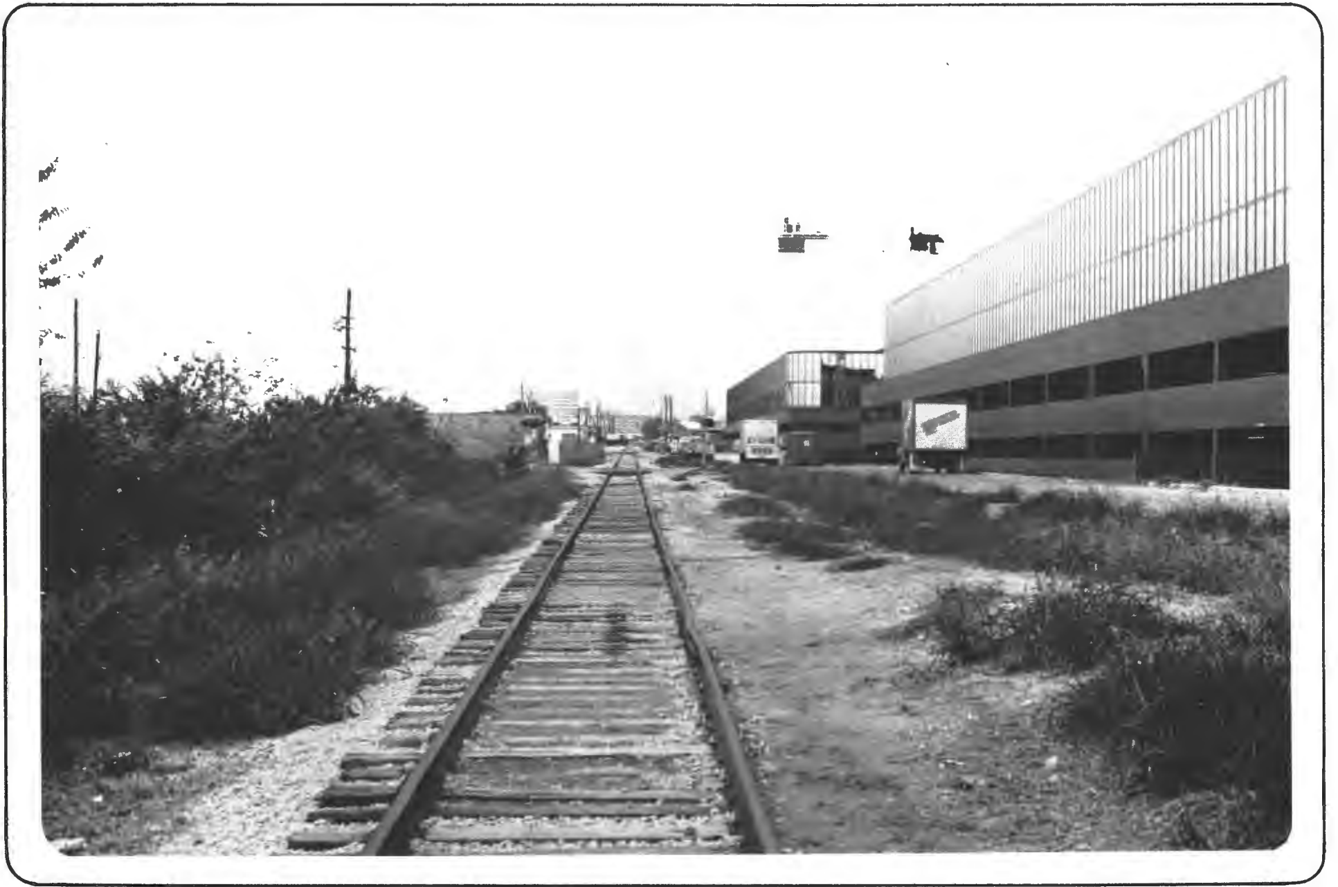
Figure 4.9 View of Rail Portion of North Central Corridor
