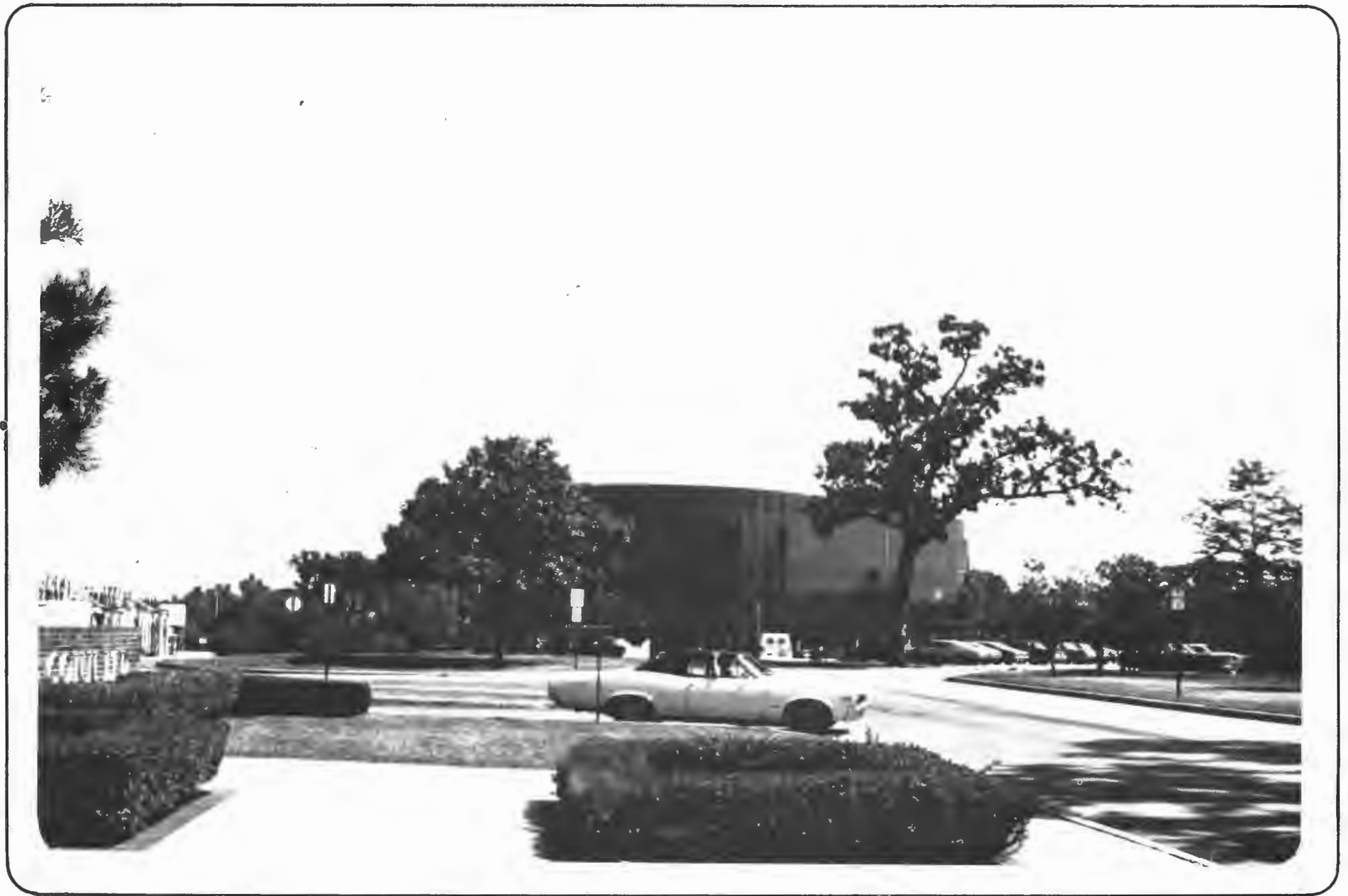
Figure 2.23 View of Enterprise Drive
