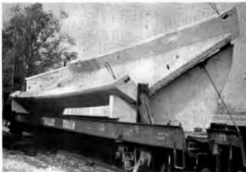
FIGURE 2.1.33. GUIDEWAY PREFABRICATION SECTION OF THE BRADLEY AIRPORT SYSTEM.
