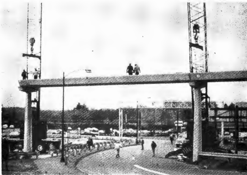
FIGURE 2.1.32. GUIDEWAY PREFABRICATION SECTION OF BRADLEY SYSTEM
