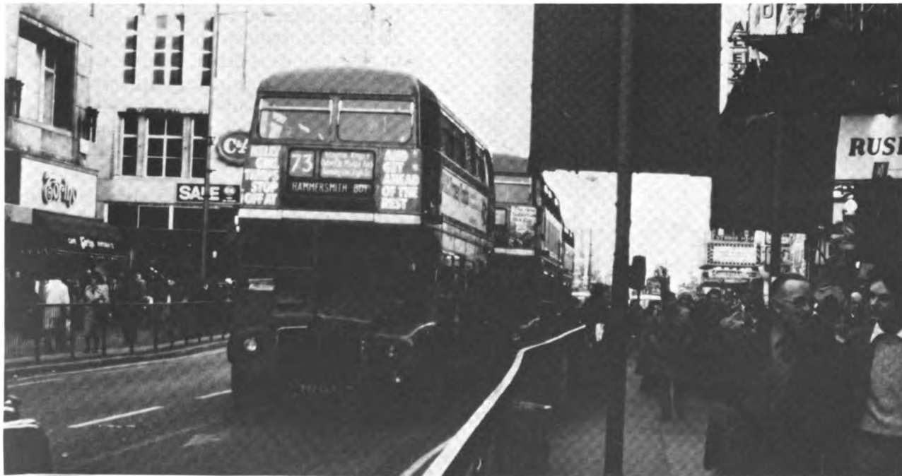
Oxford Street Transit Mall
