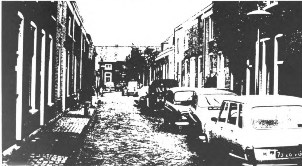
Delft: Residential Street Before Construction of a Woonerf
