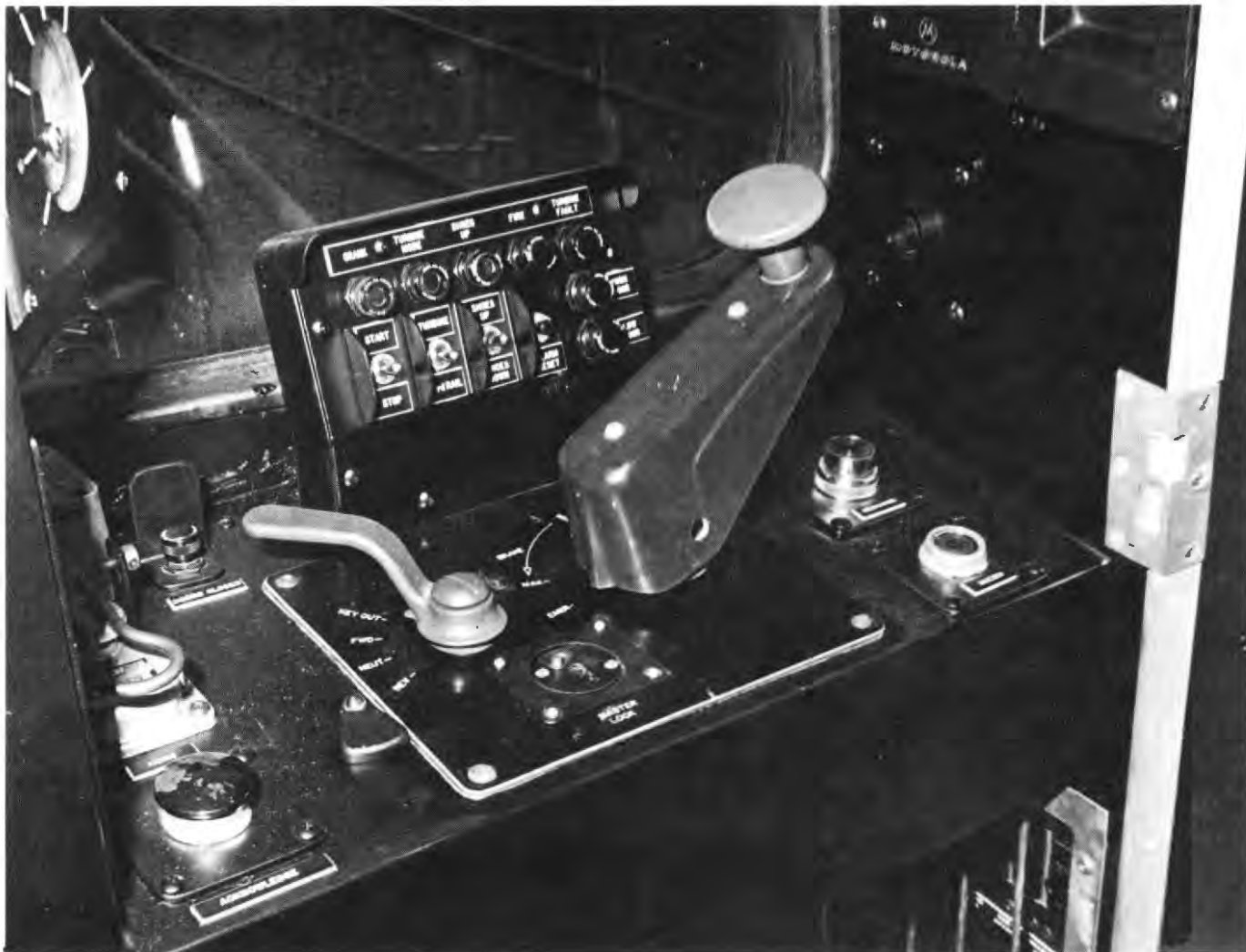
Figure 1.4-7 Engineman's Turbine Control Panel
