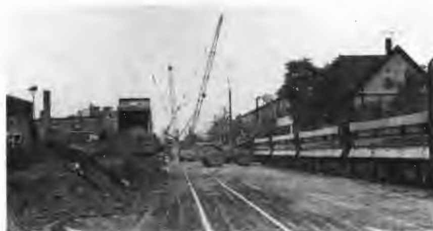
Figure 5 Muck Train Loading Area.
