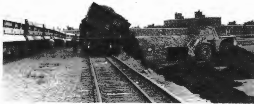
Figure 4 Side Dumping of Muck at End of Spur Line.
