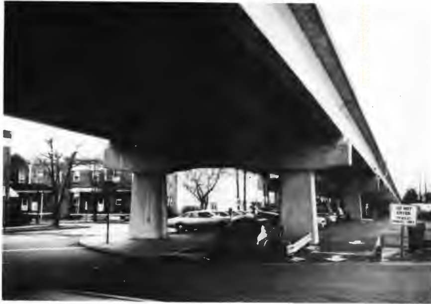
FIGURE 7. PATCO ELEVATED SITE FOR NOISE MEASUREMENT (TYPICAL CONSTRUCTION)
