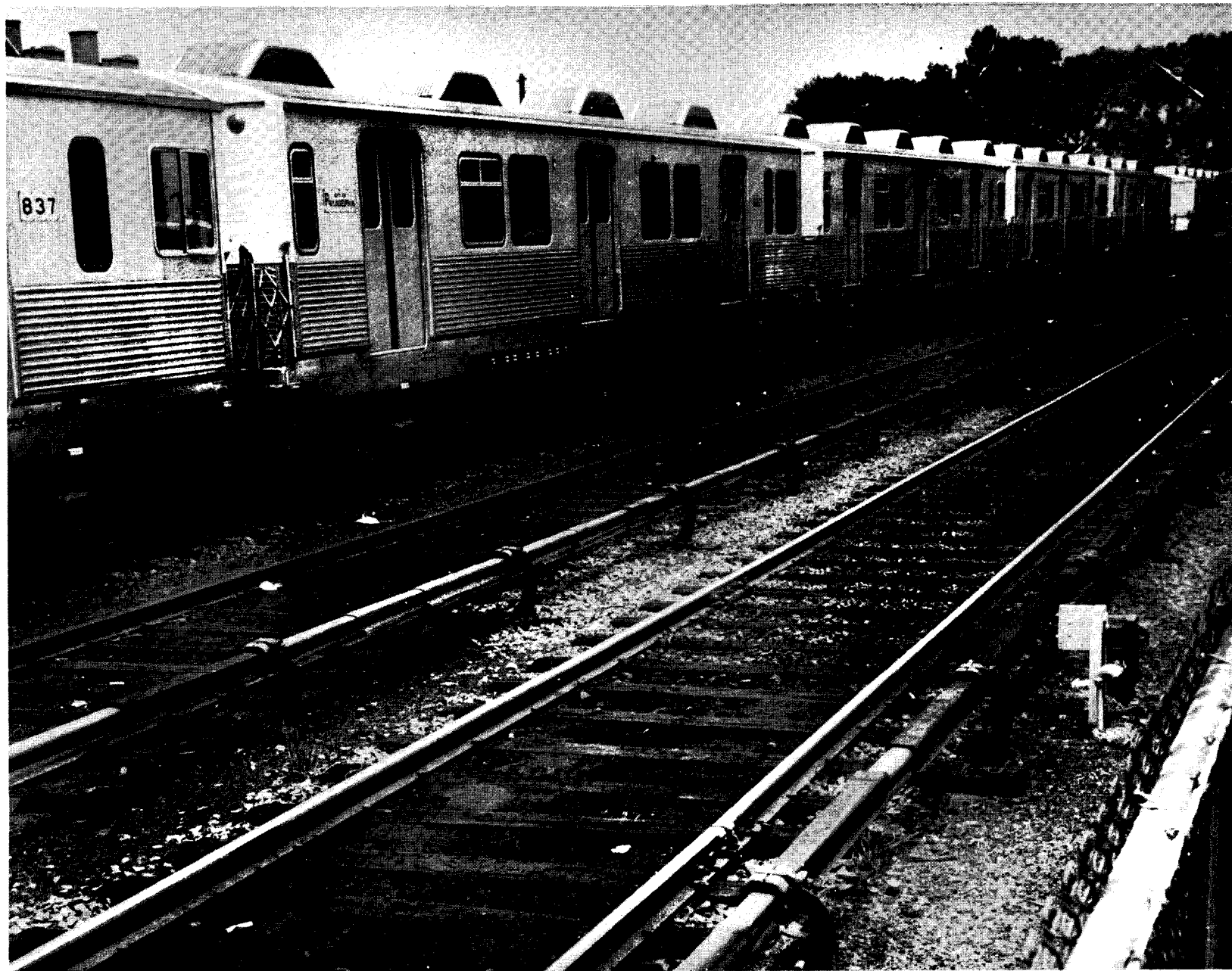
Figure 43. Southeastern Pennsylvania Transportation Authority - Market-Frankford Subway Elevated Line
