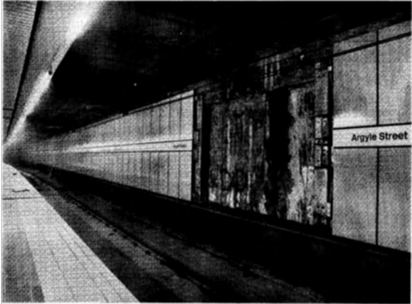
FIGURE 8 VIEW OF STATION NEARING COMPLETION SHOWING THE DECORATIVE LINING PANELS.
