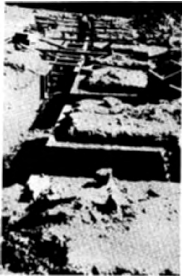
FIGURE 2 T SHAPED GUIDEWALLS
