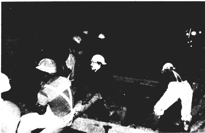
FIGURE 62. TUNNEL CONCRETING OPERATIONS
