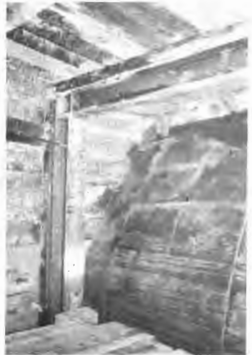
FIGURE 92. INTERSECTION WITH STEEL LINER.
