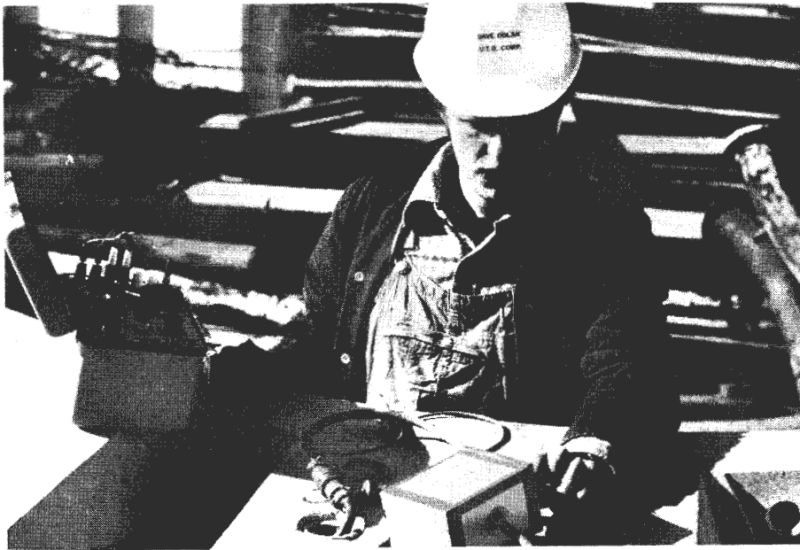
FIGURE 11. CHECKING OUT IMBEDDED STRAIN GAGES IN CONTRACTOR'S YARD
