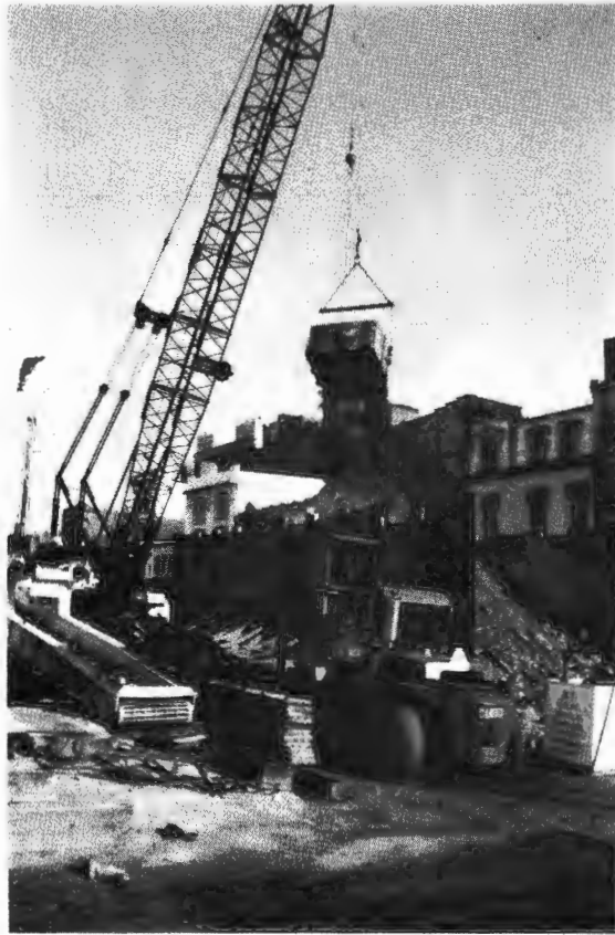
FIGURE 59. MUCK CAR BEING DUMPED INTO BIN
