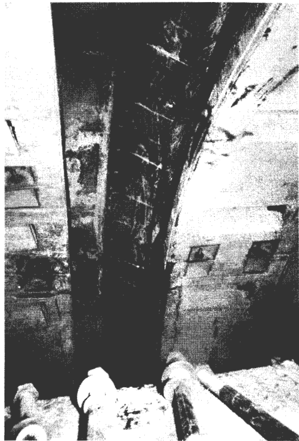
FIGURE 80. PHOTO OF INSTALLED SEAL
