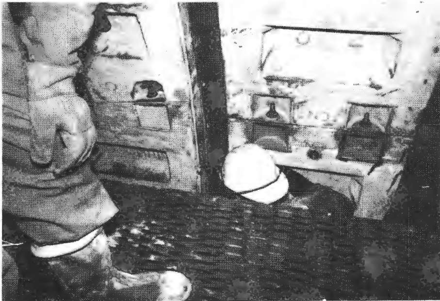
FIGURE 86. PUSHING ASSEMBLED RING BACK TO CONNECT WITH PREVIOUS RING
