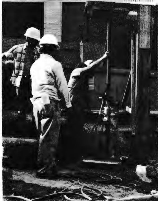
Figure VIII-3: Coring of Shotcrete Samples.
