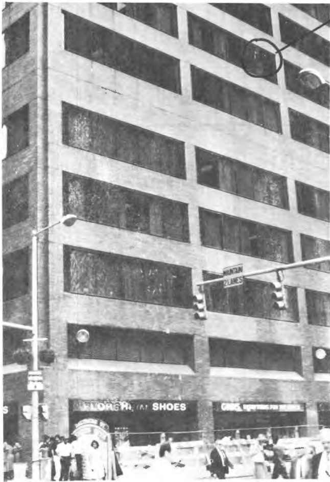
(a) Slurry Splashed Onto Face and Windows of Building From Grab bucket During Trenching Operations.
