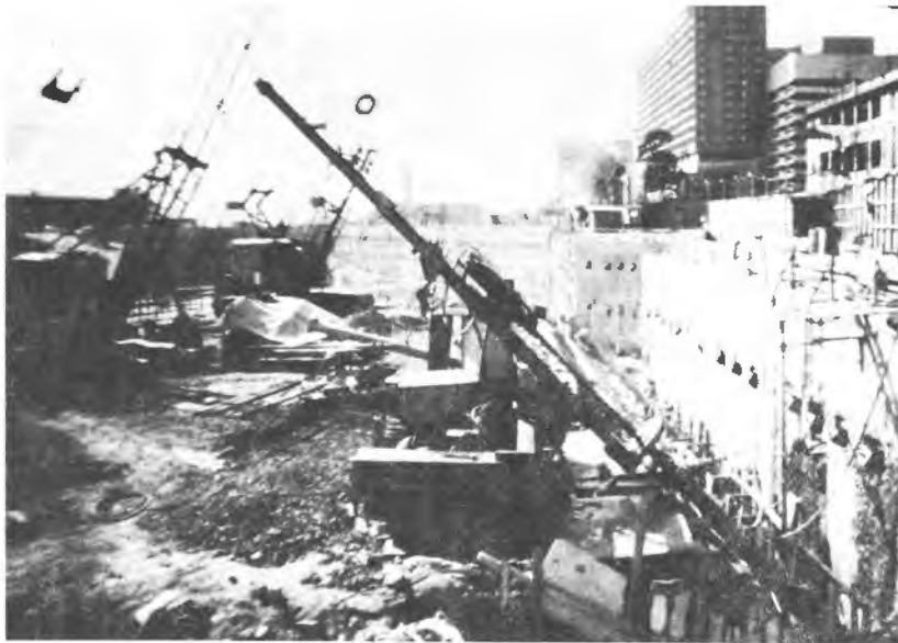
a. TYPICAL TIEBACK INSTALLATION (PHOTO COURTESY OF ICOS)
