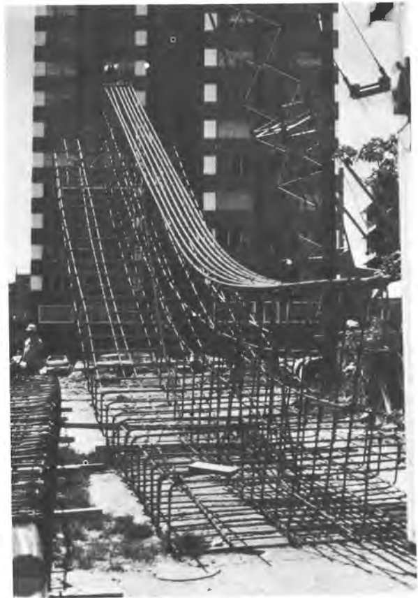
Figure 58. T Shaped Reinforcing Cage
