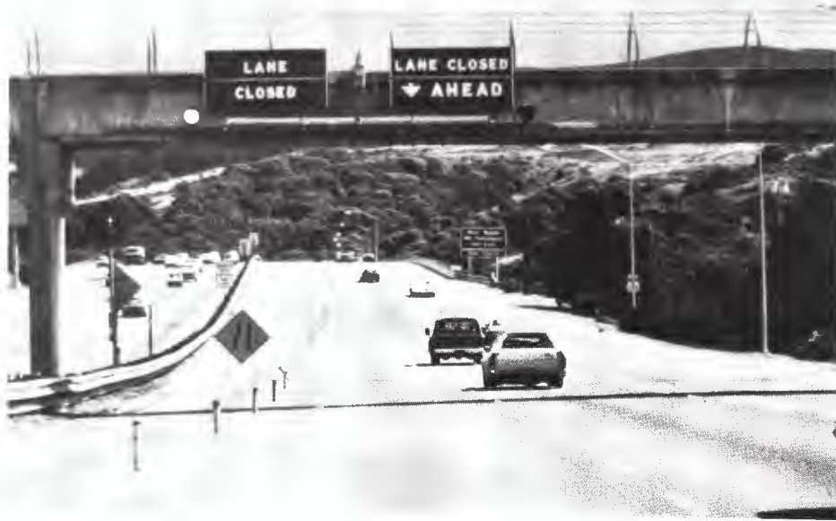
Figure 4-13. Transition on Contraflow Lane (U.S. 101; San Francisco, CA)
