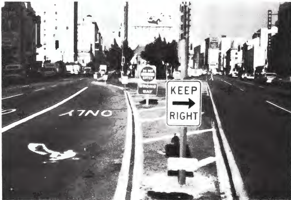
Figure 4-14. Contraflow Transition on Surface Street (Spring Street; Los Angeles, CA)
