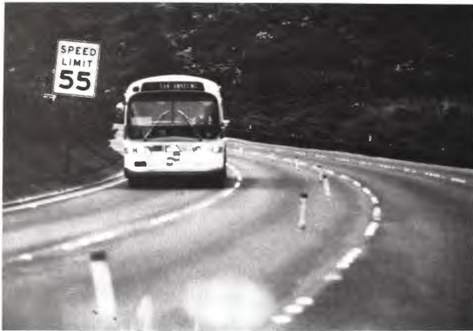
Figure 4-1. Buffer Lane - U.S. 101 (San Francisco Bay Area)
