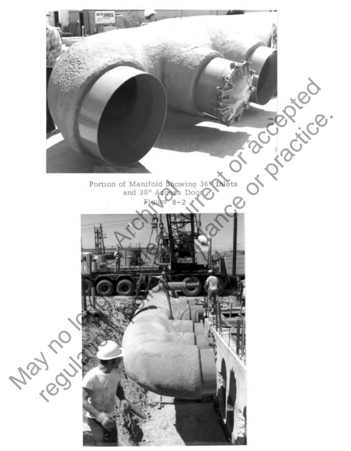
Installation of Manifold Figure 8-3 the station, and its performance is expressed as the required discharge in gallons per minute at the resulting total dynamic head. The efficiency of a stormwater pump at its design point may be 75 or 80% or even more, but this will depend on the type of pump.
