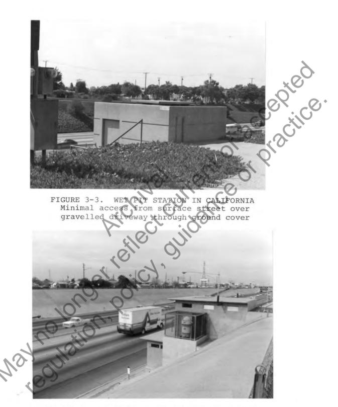
FIGURE 3-4. POORLY SITED STATION IN ARIZONA Original construction was adjacent to freeway pavement at low point. Subsequent retro-fit provided access from frontage road aesthetics, but in most cases the utility company can at best only provide service from high voltage lines on adjacent poles, thence underground to the station. Sometimes the service is overhead to the station, with hazard to crane service for handling equipment. Overhead service should be avoided if possible.
