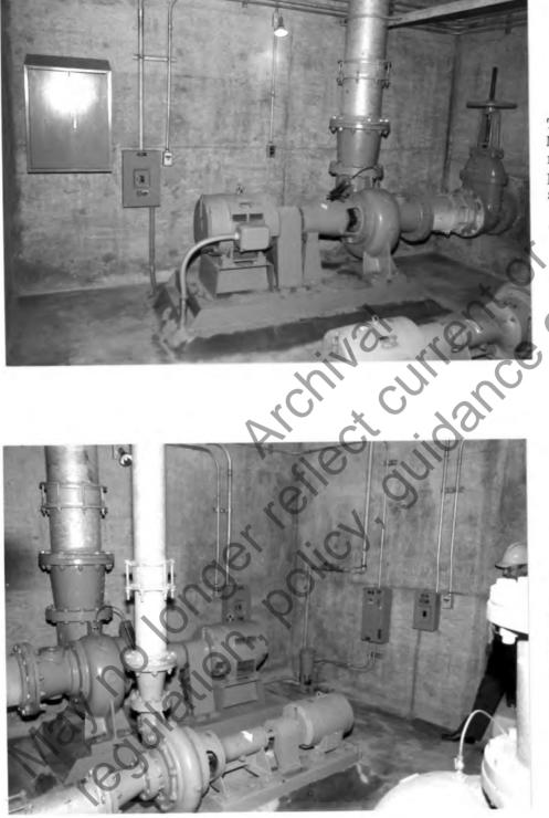
FIGURE 10-Typical Horizontal Motor (25 HP) for non-clog horizontal pump in dry-pit station. Los Angeles, CA (See Figures 3-1 and 3-2)
