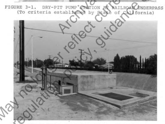
FIGURE 3-2. SAME STATION AS FIGURE 3-1 Relationship of wet-well to dry-pit, access to station and electrical service underground to meter box can all be observed. In the case of small stations with submersible pumps, the wetwell can reasonably be at the low point, provided the electrical control panel is located on higher ground. See Figures 2-26 and 2-27. Inlet gratings can be as observed in Figure 3-1.
