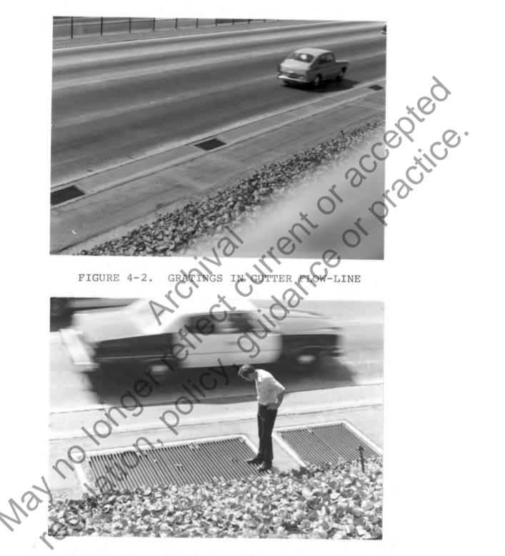
FIGURE 4-3. ACCESS GRATING TO STORAGE BOX Note location in shoulder and relationship to gutter flow-line
