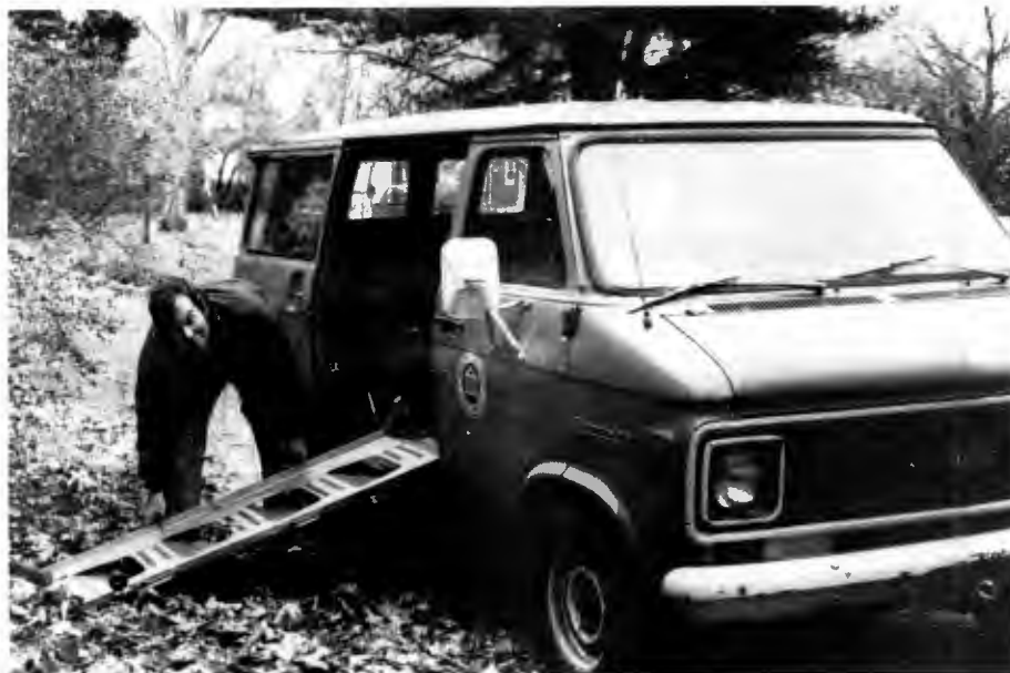
A TRADE van equipped with wheelchair ramp. (photo: D. Fleishman)
