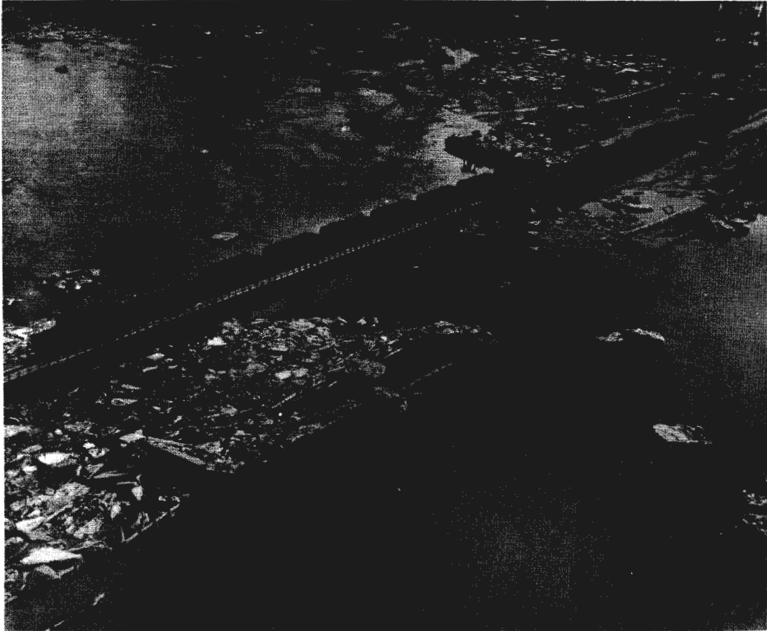
Figure 15. Photo taken about one month after the 1964 earthquake. Highway and railroad bridges across Twentymile River, 48 miles southeast of Anchorage, Alaska. Railroad cars were left on the bridge to help stabilize the structure during high tides. (Photo courtesy of U.S.D.A. Forest Service)
