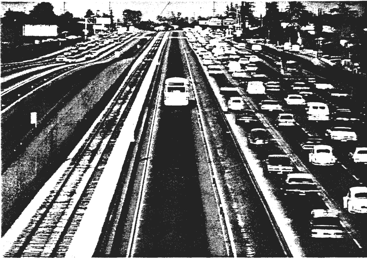
Separate HOV Facility Los Angeles, California
