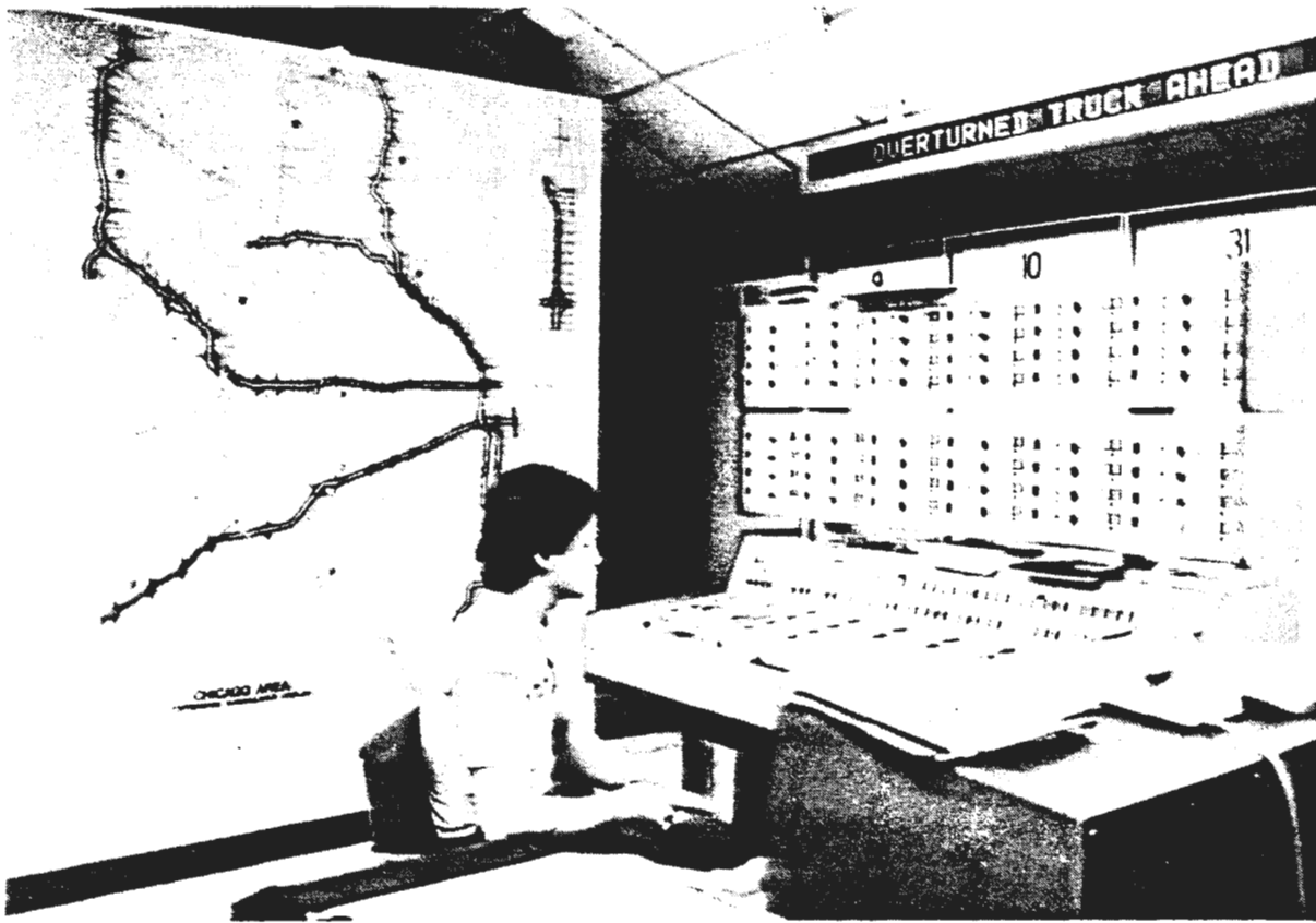
Traffic Control Center Chicago, Illinois
