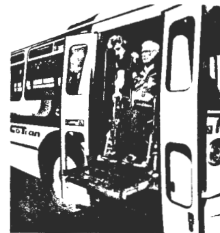
Ramp is raised by bus driver.
