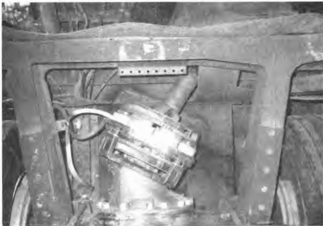
870 GRUMMAN FLXIBLE AFTER TELMA RETARDER HAS BEEN INSTALLED FIG. 4.12
