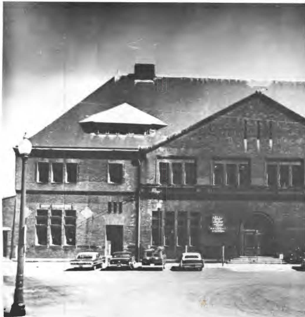
New London's Union Station, before and after its restoration.
