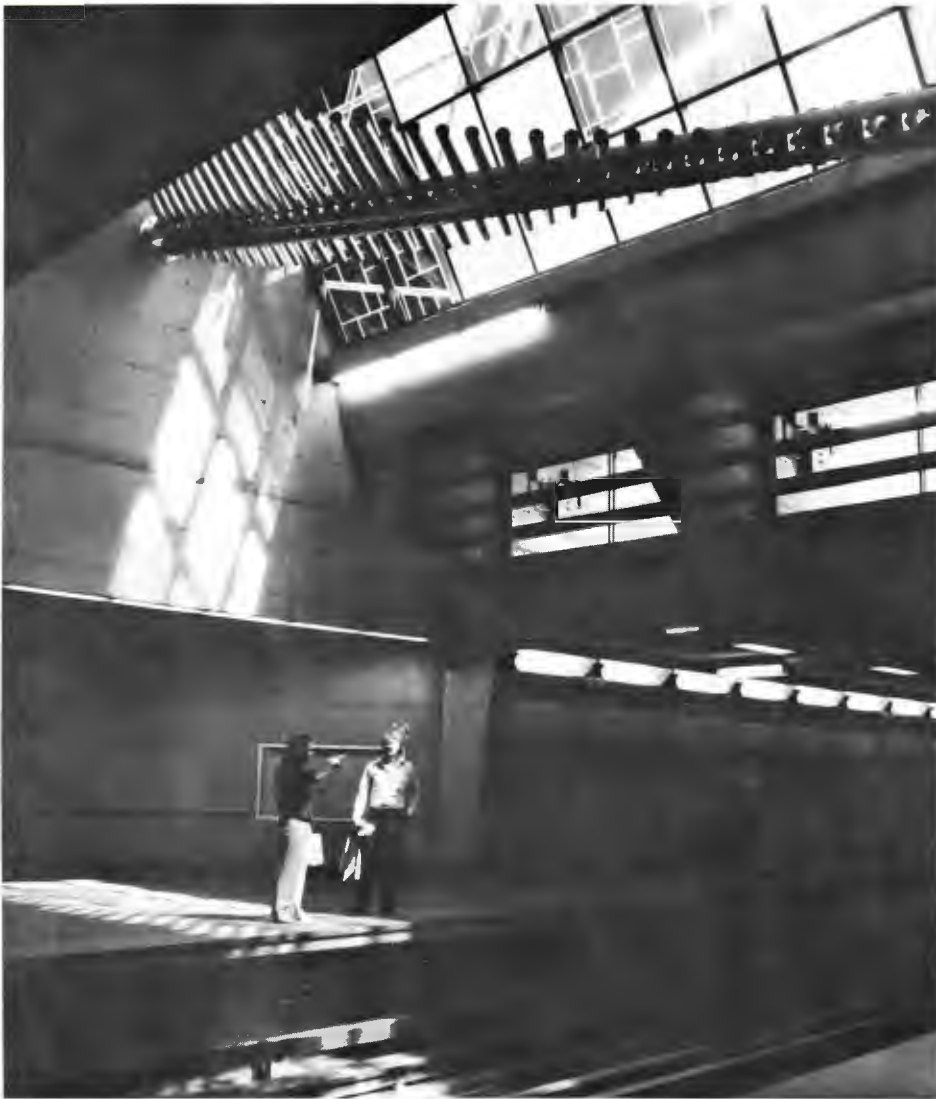
Skylights brighten the Vendome station.
