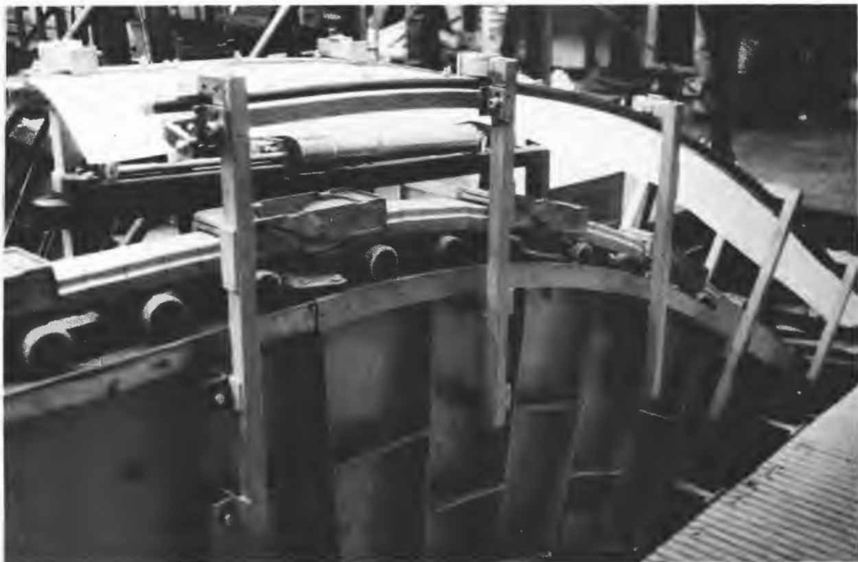
TRAX AWS - Photo of handrail entry with protective cover and balustrade removed. Cylinder and plunger is automatic shutdown device in event of entrapment.
