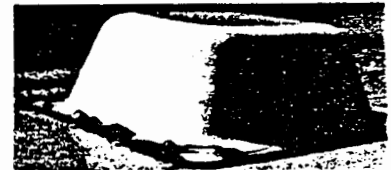
Many low powered communications sites chosen rather than one high-powered one: localized coverage eliminates poor reception. Low power enables the same frequencies to be used a short distance away. This radio antenna is located at Wilson Division, the site of C.I.S.
