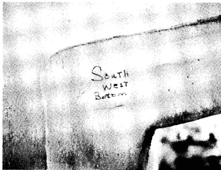
Lamellar Tear in the Compression Flange Midthickness
