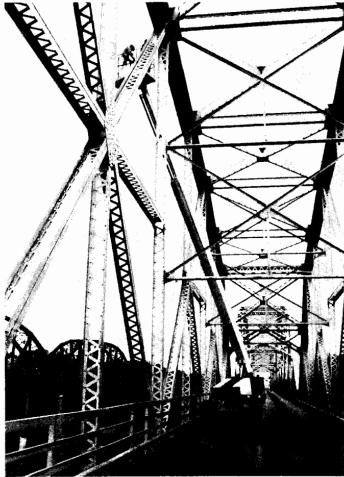
Used from bridge deck to inspect through Truss
