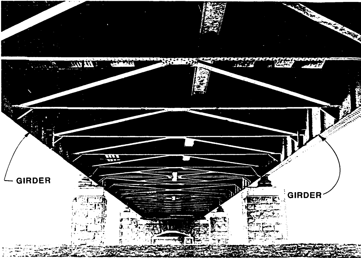
Lateral bracing system on steel two-girder bridge.
