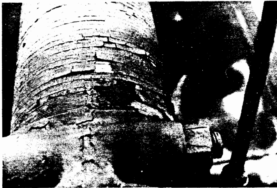
More Extensive Paint Deterioration on Cable Wrapping: Maysville Bridge (1983).
