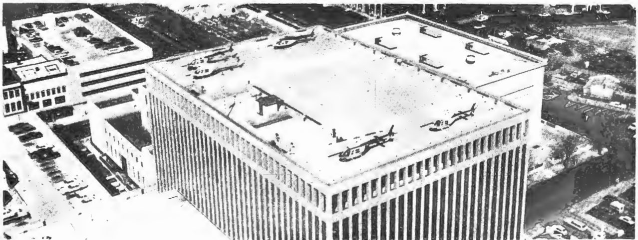
ROOFTOP HELIPORT, BALTIMORE, MARYLAND, POLICE DEPARTMENT
