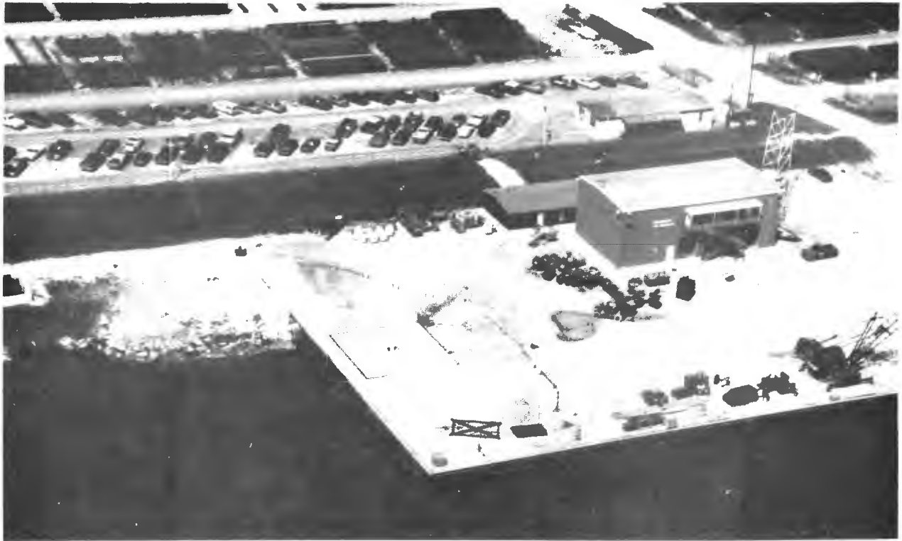
MARATHON OIL COMPANY HELIPORT, BERWICK, LOUISIANA
