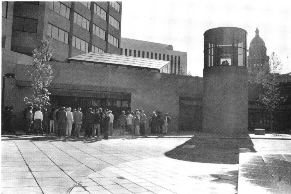
Civic Center Transfer Station in Denver at one end of the 16th Street Mall. The State Capital is in the background.
