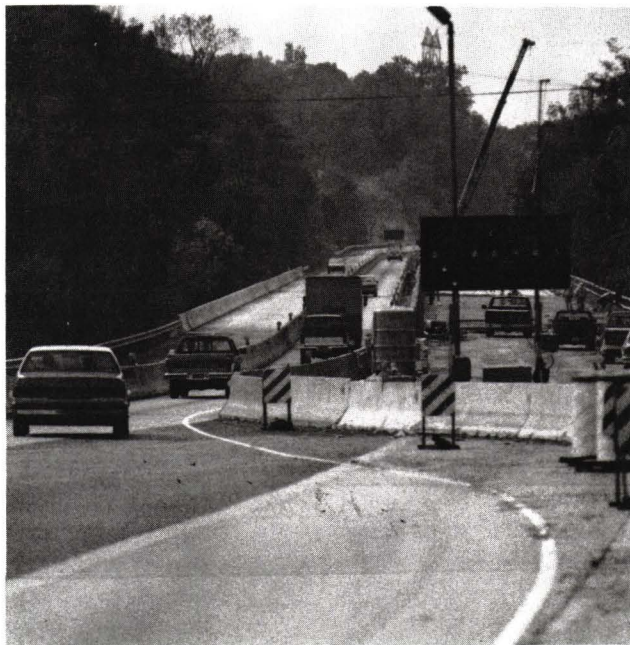
Figure 20. Application of the arrow panel in crossovers
