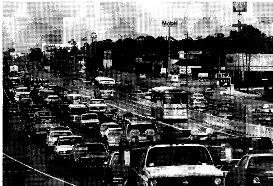
Figure 4. Transitway in Median of Katy Freeway
