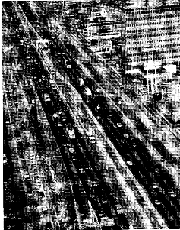
Figure 6. Slip Ramp for Transitway Access/Egress on Katy Freeway
