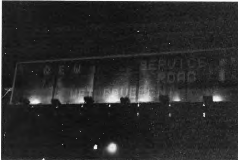
Figure 2-22. Detail of Lighting Problem With Anti-Glare Lexan (Ref. 5)
