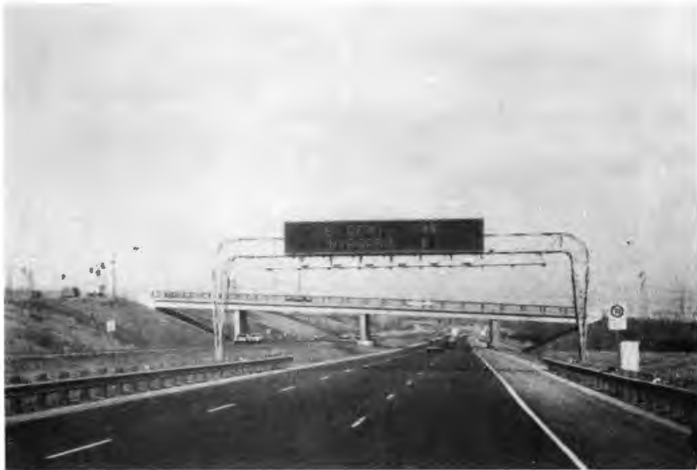
Figure 2-16. Sun in Front of Reflective Disk Sign Gives Good Visibility (Ref. 5)
