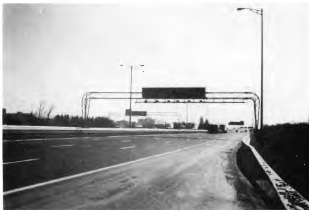
Figure 2-17. Sun Behind Reflective Disk Sign Gives Poor Visibility (Ref. 5)
