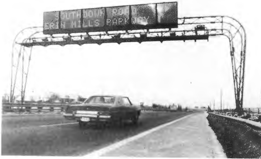
Figure 2-19. Extraneous Reflections Using Lexan (Ref. 5)
