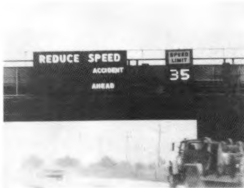
Figure 2-4. Neon-Type Blank-Out Hazard Warning and Bulb Matrix Speed Signs on the New Jersey Turnpike
