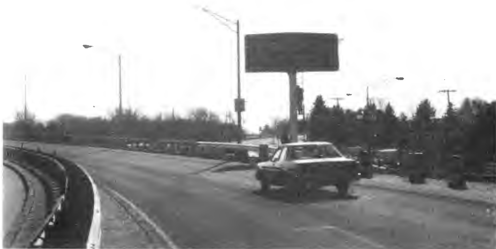
Figure 2-43. Shuttered Fiber Optic Sign in Sun (Ref. 5)
