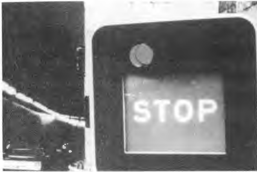
Figure 2-6. Scroll Sign Mounted Used at the Portal of the Lincoln Tunnel in New York
