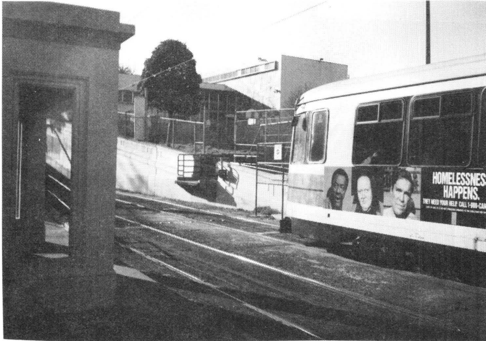
FIGURE 2-13. MUNI TRAIN MAKING NORMAL STOP SHORT OF MINI-PLATFORM
