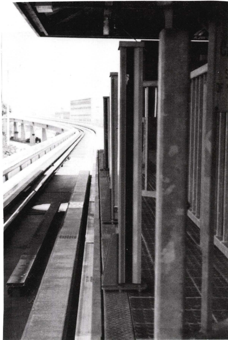
FIGURE 3-27. PILLAR WITH ROW OF FOUR INFRARED DETECTORS
