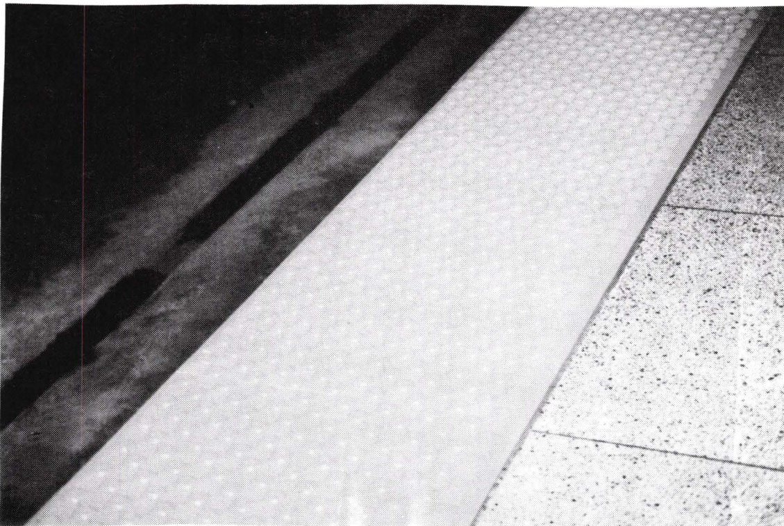
FIGURE 3-8. "ARMOUR-TILE" INSTALLED AT TRANSIT PLATFORM EDGE
