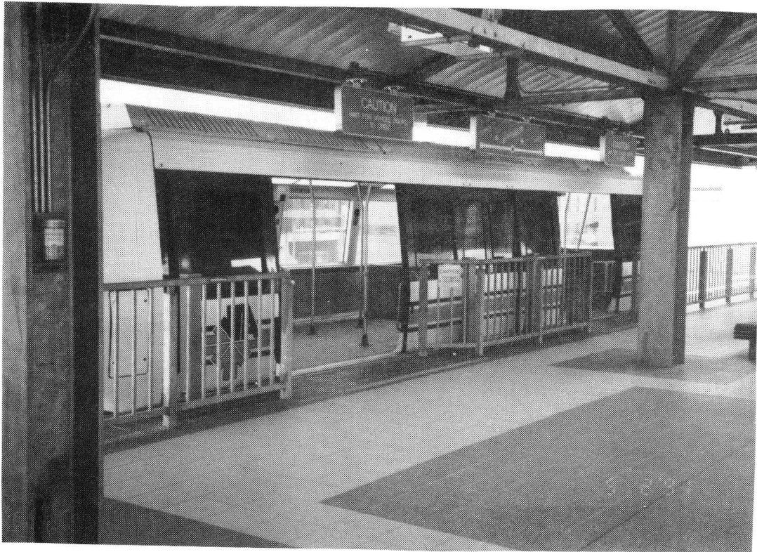
FIGURE 3-26. JACKSONVILLE STATION WITH RAILING SET BACK TWO FEET FROM PLATFORM EDGE
