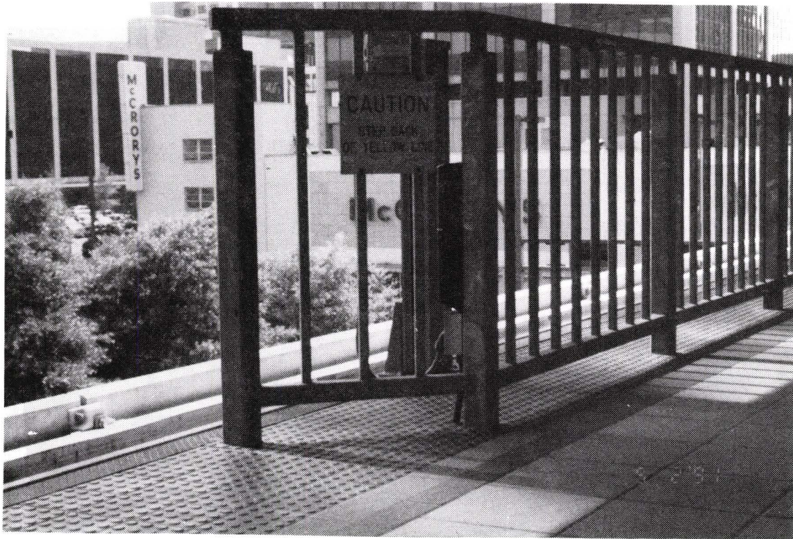
FIGURE 3-14. AMERICAN OLEAN WARNING TILE IN JACKSONVILLE, FLORIDA
