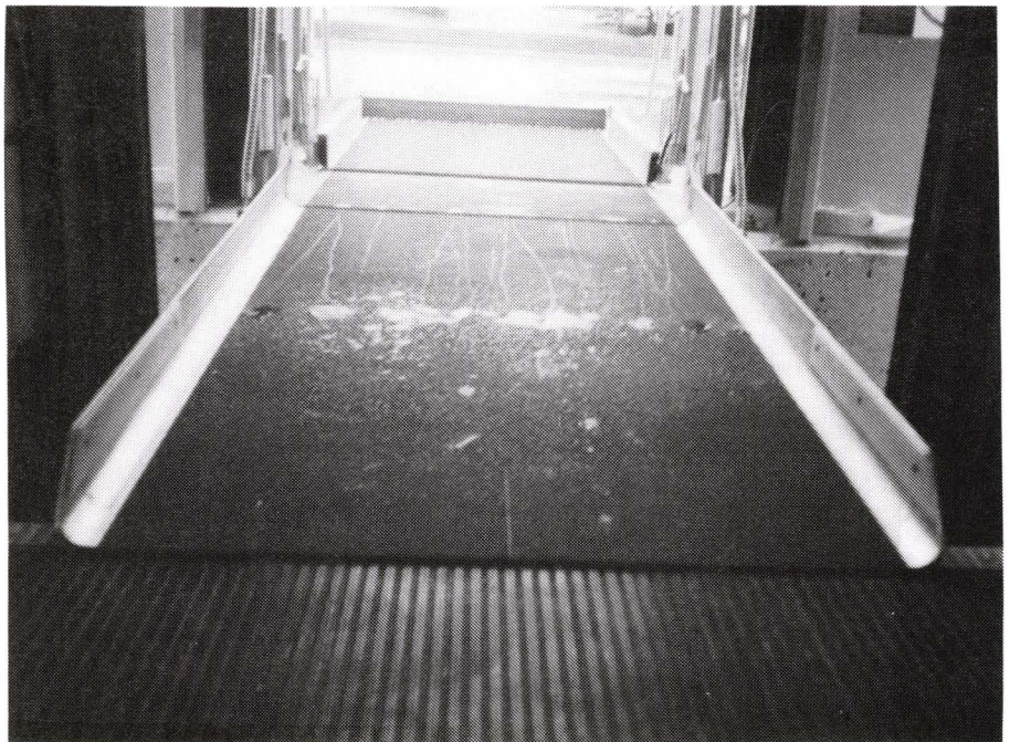
FIGURE 2-25 FULLY DEPLOYED SANTA CLARA LIFT IN RAISED POSITION → PROVIDES CONTINUOUS “GANGPLANK” ONTO LIGHT RAIL CAR
