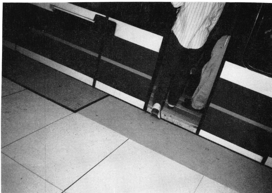
FIGURE 3-16. SERVICE TEST OF WAFFLE PATTERN RUBBER TILE (LEFT SIDE) AND NON-SKID ALUMINUM OXIDE (RIGHT SIDE) AT MUNI VAN NESS STATION
