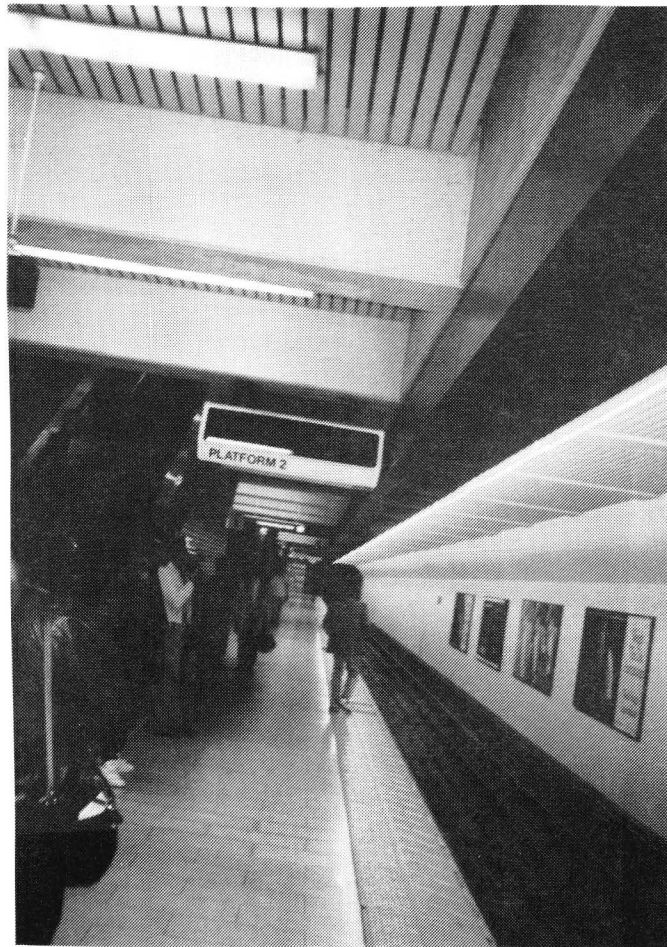
FIGURE 3-17. PERSON USING BART WARNING STRIP AS WALKWAY
