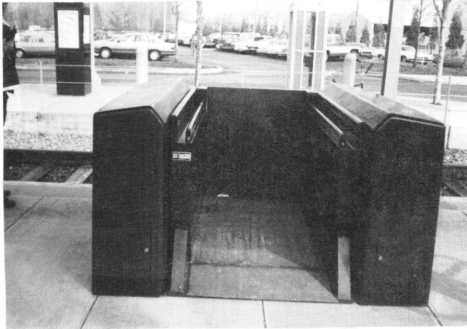
FIGURE 2-29. NORMAL LOWERED POSITION OF PORTLAND LIFT
