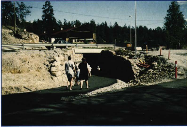
In rural Akershus county, the high-type construction and quality of materials used in this ped/bike underpass point out the importance of pedestrian and bicycle travel in Norway.
