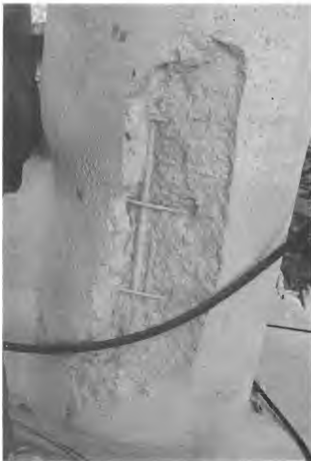
FIGURE 2 Sprayed zinc concrete surface.
