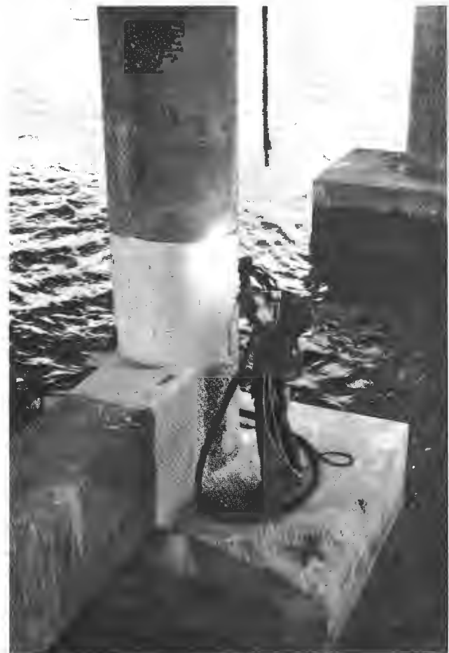
FIGURE 1 Application of zinc anode.
